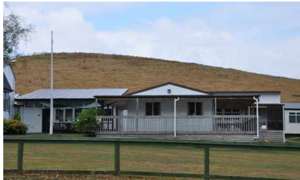
Photo 50. Well respected school within the Ngaruawahia area
