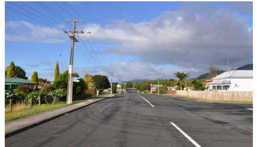
Photo 32. Pedestrian facilities are limited throughout the town
