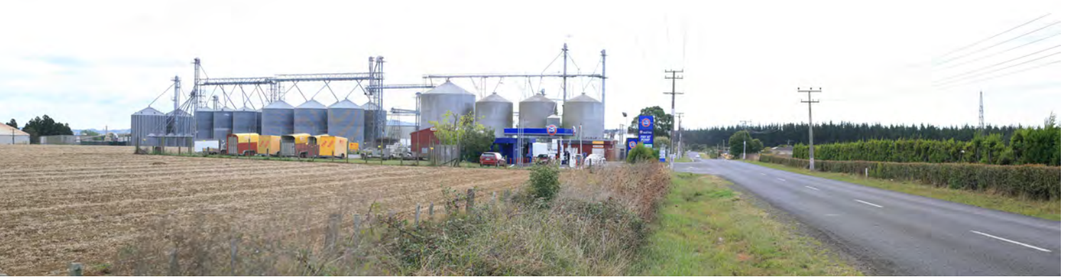
Bollard Road, looking northwest
