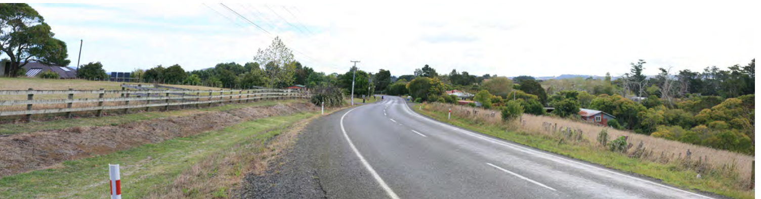
Whangarata Road, looking west
