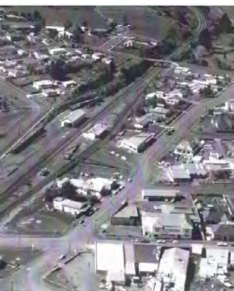
Railway and Tuakua Township A
