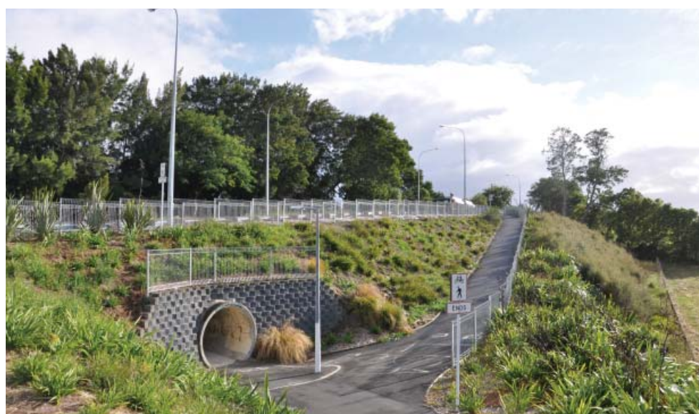
Photo 17. Pedestrian and cyclist routes are affected by the by-pass
