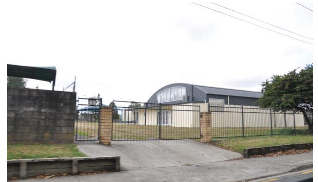
Photo 33. Horotiu Primary School
