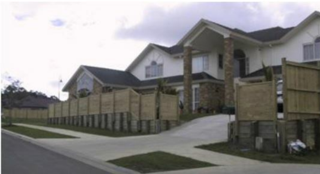
Figure 31: Retaining walls detract from streetscapes
