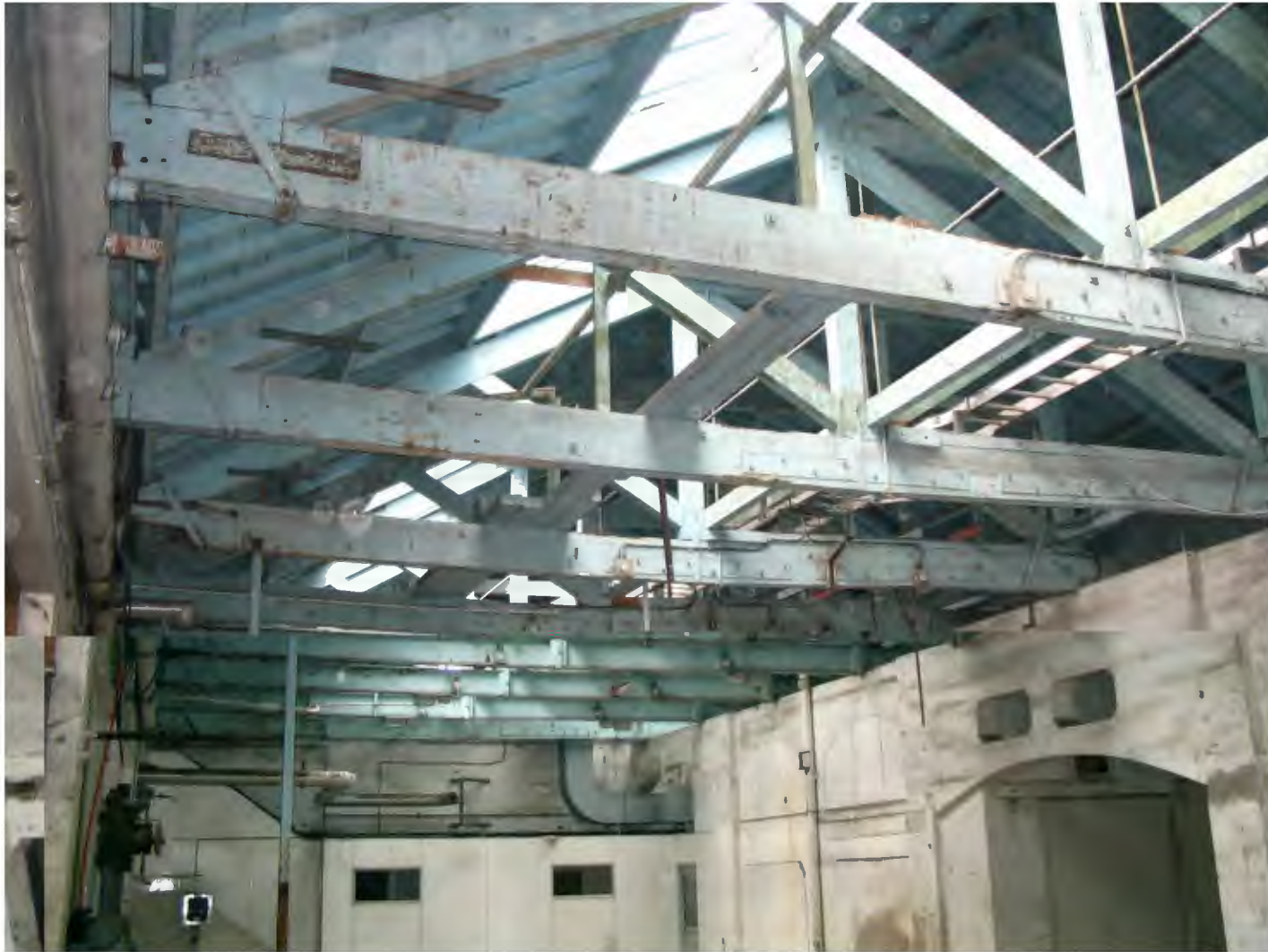
Kauri sarking & Rimu trusses in The Glaxo Building
