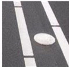
Diagram 1: Examples of rumble strips or markers between footpaths and cycle paths
