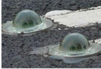
Diagram 1: Examples of rumble strips or markers between footpaths and cycle paths
