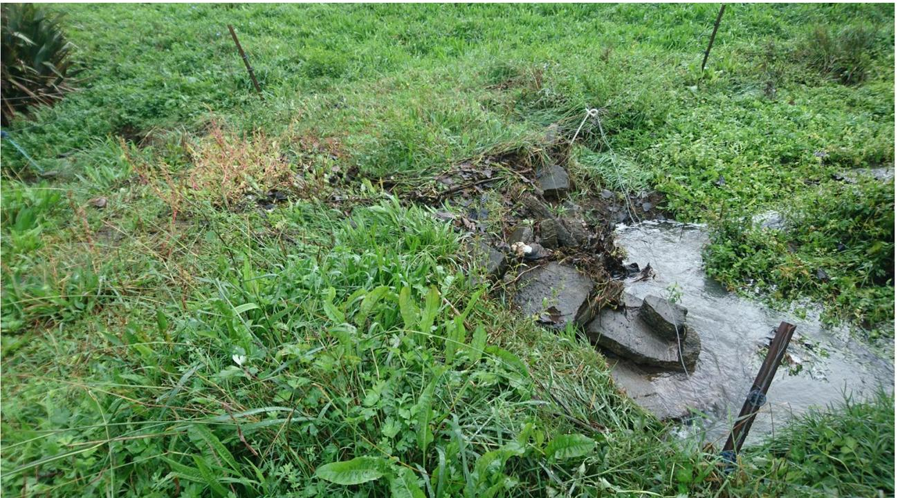
Upper side vehicle, stock culvert crossing not coping with storm water volume. Photo ref: DSC\_0849 10 May 2023.
