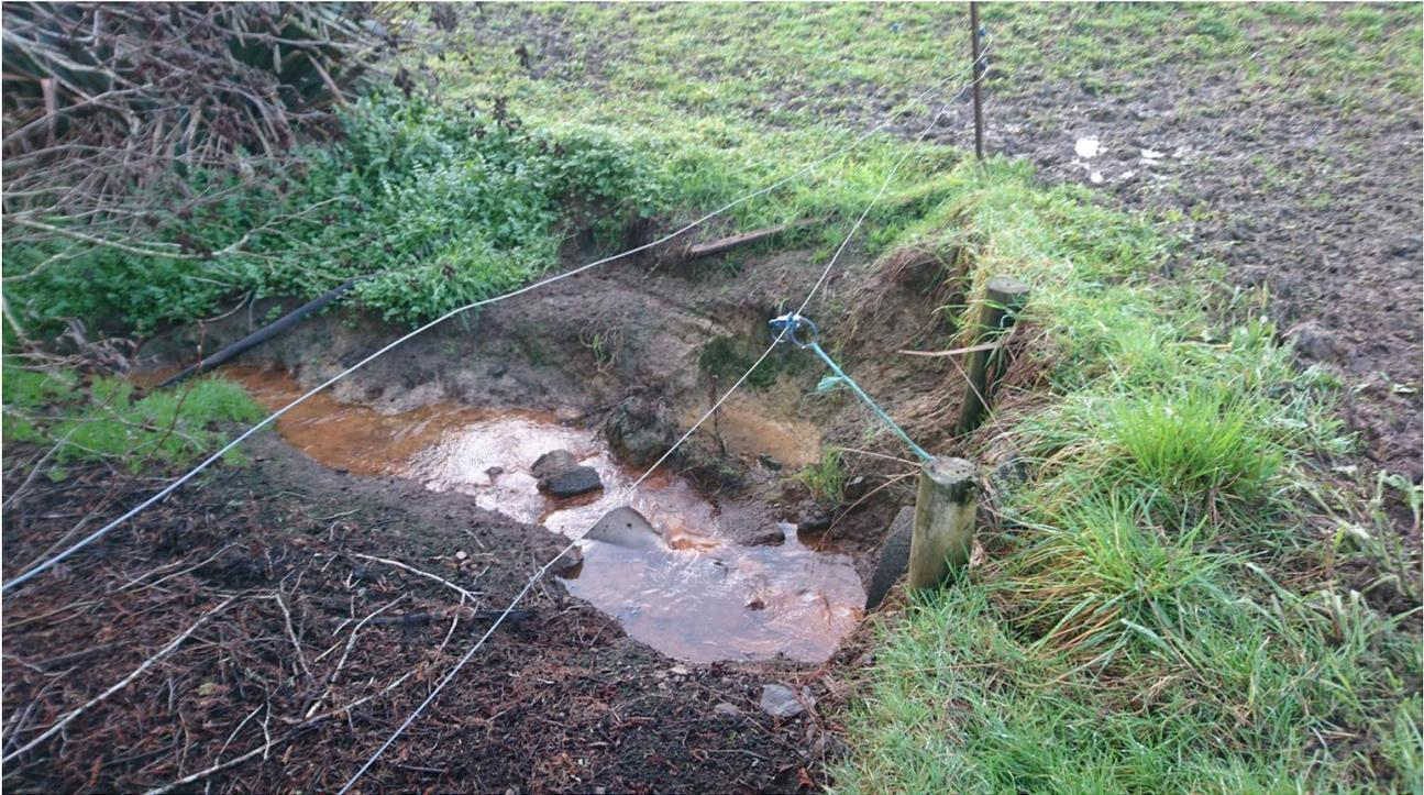
Lower side vehicle, stock culvert crossing showing erosion. Photo ref: DSC\_1217 17 June 2023.
