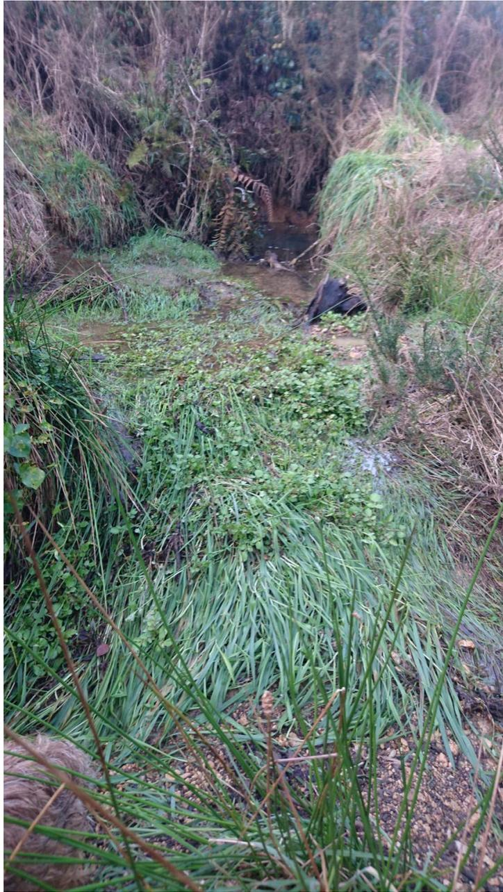
D1 discharge showing erosion and clay stone sediment above NIMT #1 culvert. Photo ref: DSC\_0938 13 May 2023.
