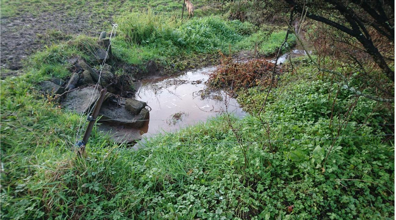
Upper side vehicle, stock culvert crossing showing erosion. Photo ref: DSC\_1215 17 June 2023.
