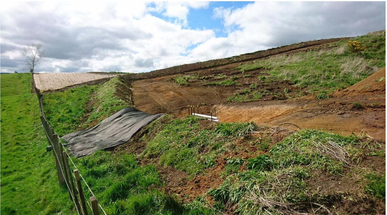
Stage 5 discharge 1 pipe and construction of discharge point onto my land. Photo ref: DSC\_0480\_1 2 October 2021.
