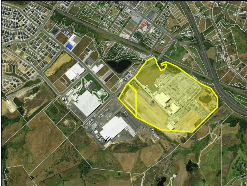
Figure 1 Aerial Photo of Hynds Factory Site (source: GRIP)
