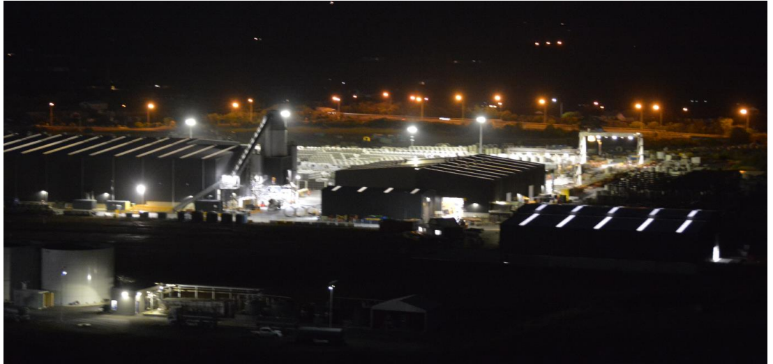
Figure 5 Photo looking north, showing:
