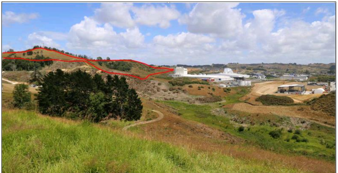
Figure 7 Photo looking south west from the 62 Bluff Road site (refer Boffa Miskell viewpoint 7) and showing the relationship between the hillslopes on which the HVL development will sit (indicatively outlined in red) and the Synlait and Hynds operations.
