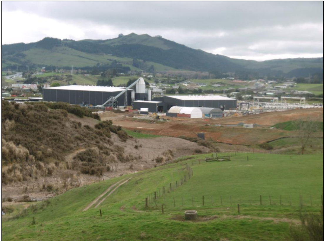
Figure 8 Photo showing batching plant (16m) and batching tower (29m). Photo is taken, by me, from 62 Bluff Road site.
