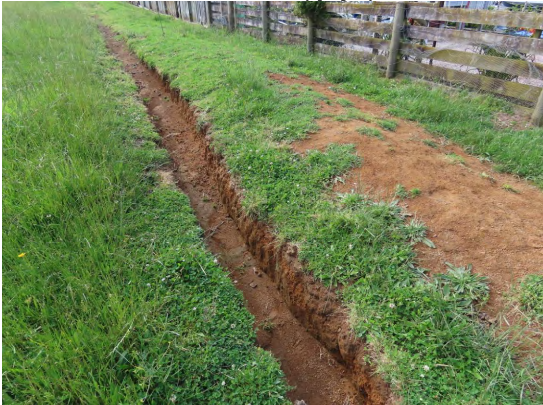
Plate 4. Small excavated drain with spoil adjacent, note the modern tantalised posts on the property border with neighbouring residential properties.
