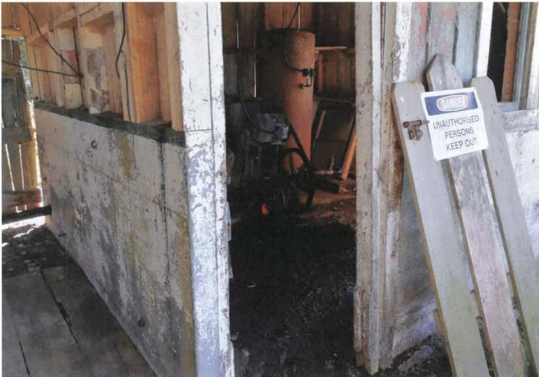
Photograph 2-3: Farm sheds with pump and aboveground storage tank. Evidence of ponded area around pump in the shed. Farm sheds are located immediately outside the property boundary of the subject site, approximately in the middle third of the site.
