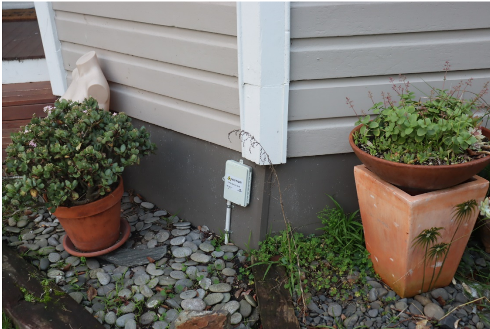
Shiplap weather boards not original
