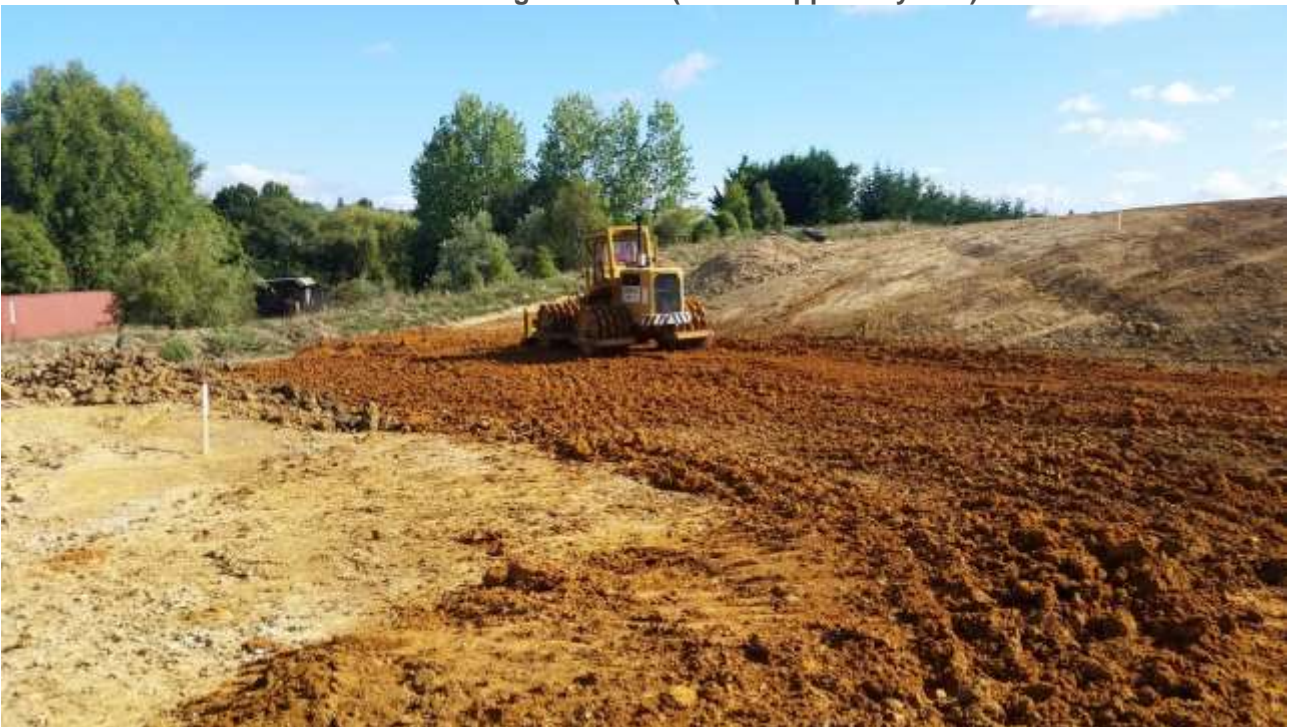
Photo 12 : Mixing of subsoil (Photo supplied by TKL)
