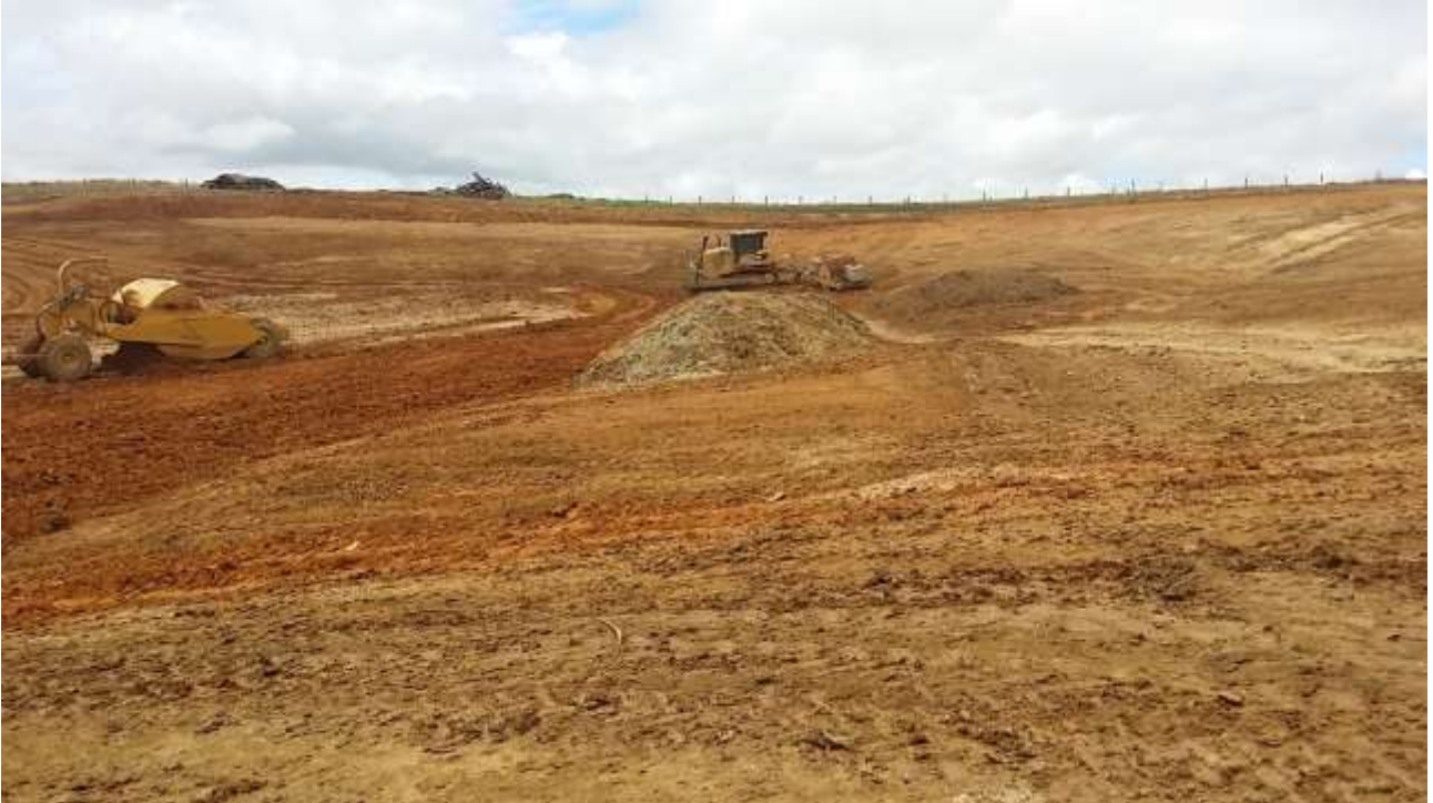
Photo 12 : Mixing of subsoil (Photo supplied by TKL)
