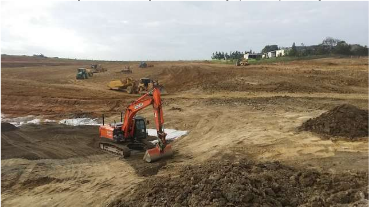
Photo 10: Mixing of subsoil (Photo supplied by TKL)
