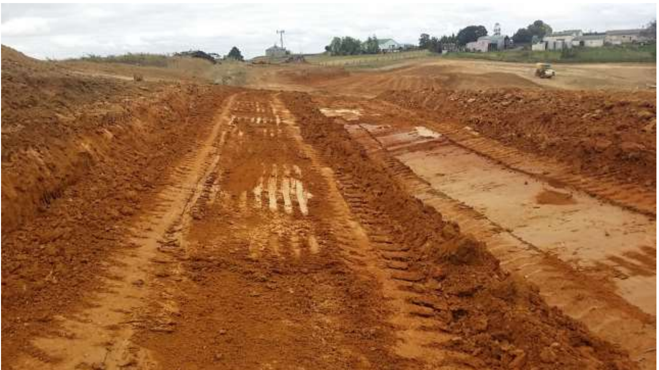
Photo 8: Mixing of the subsoils (Photo supplied by TKL)
