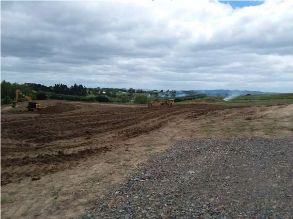
Photo 2: Mixing of topsoil
