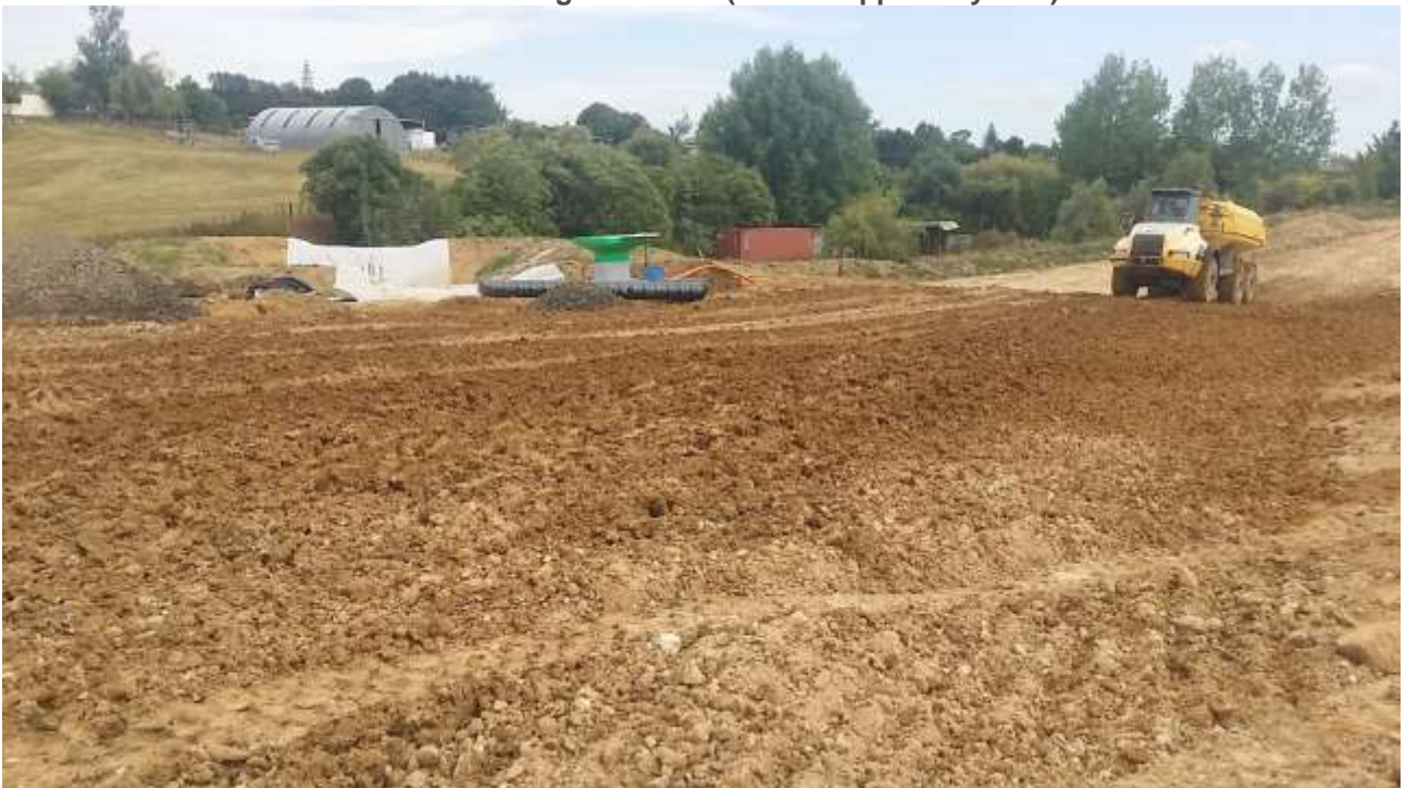
Photo 10: Mixing of subsoil (Photo supplied by TKL)
