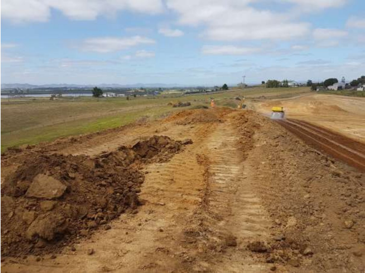
Photo 8: Mixing of the subsoils (Photo supplied by TKL)
