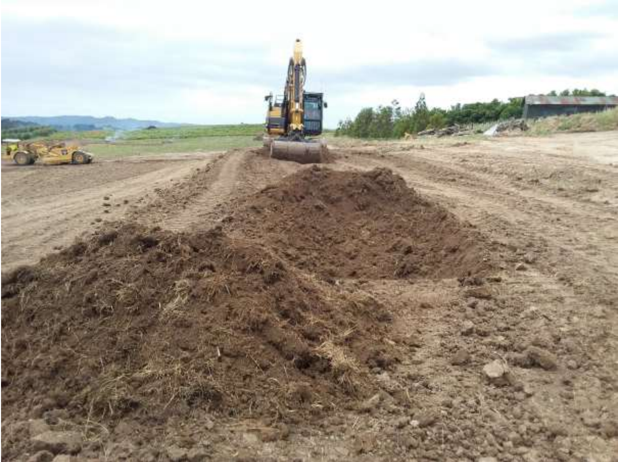
Photo 2: Mixing of topsoil
