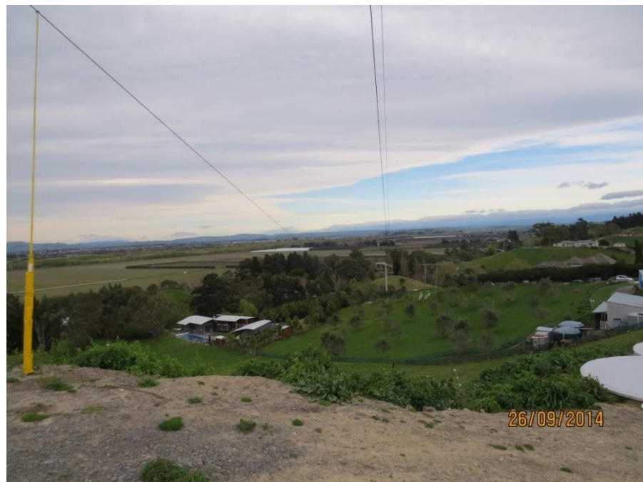
Figure 5: Hastings ground clearance violations
