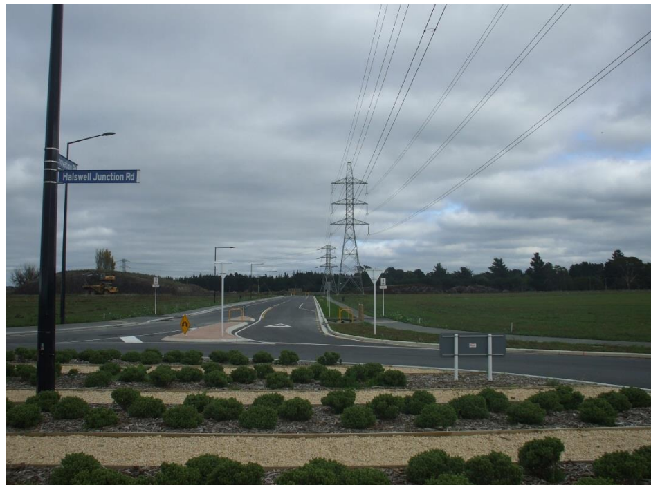
Figure 18: Waterloo Business Park
