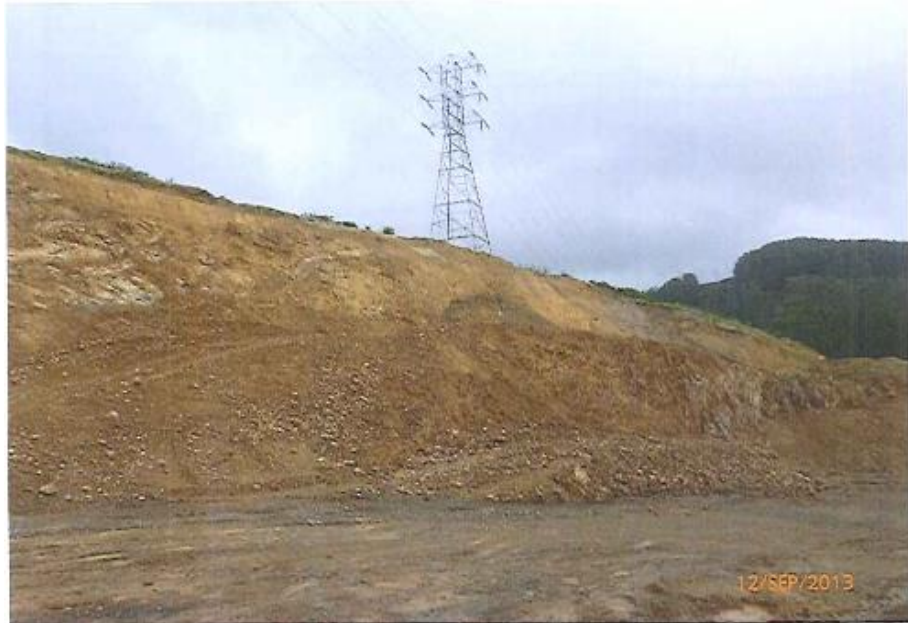
Figure 3: Earthworks in Porirua
