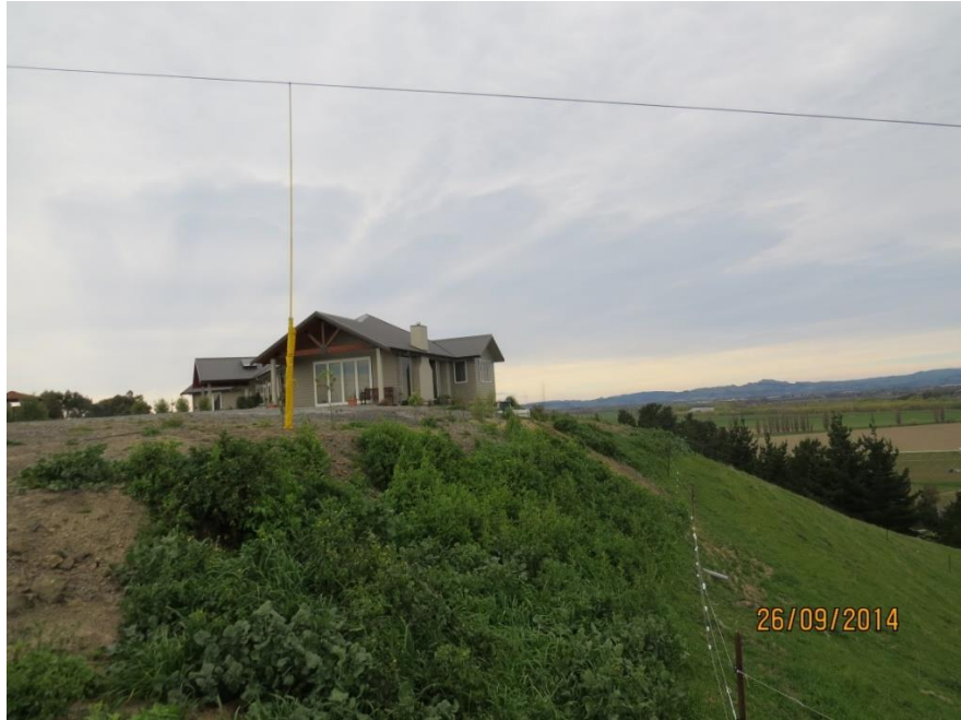
Figure 6: Hastings ground clearance violations
