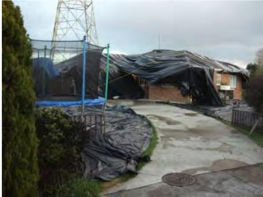
Figure 5: Tower painting in an urban setting
