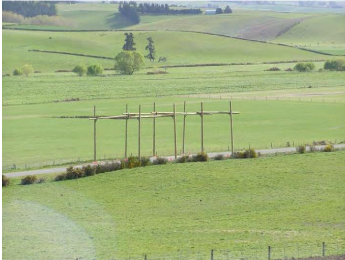
Figure 12: Typical hurdles installed to mitigate potential conductor drop during wiring
