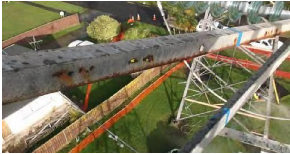
Figure 4: Tower corrosion
