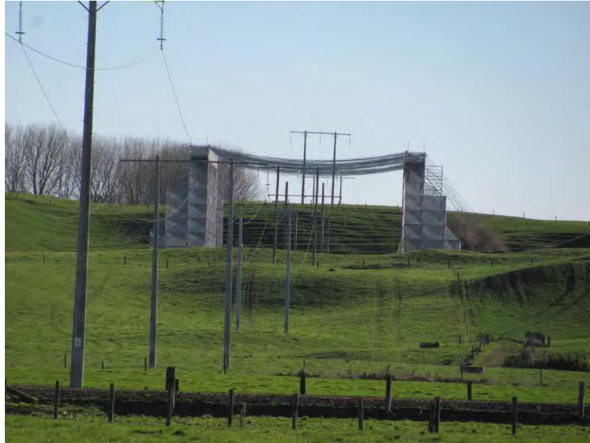
Figure 9: Scaffolding protection structure for stringing
