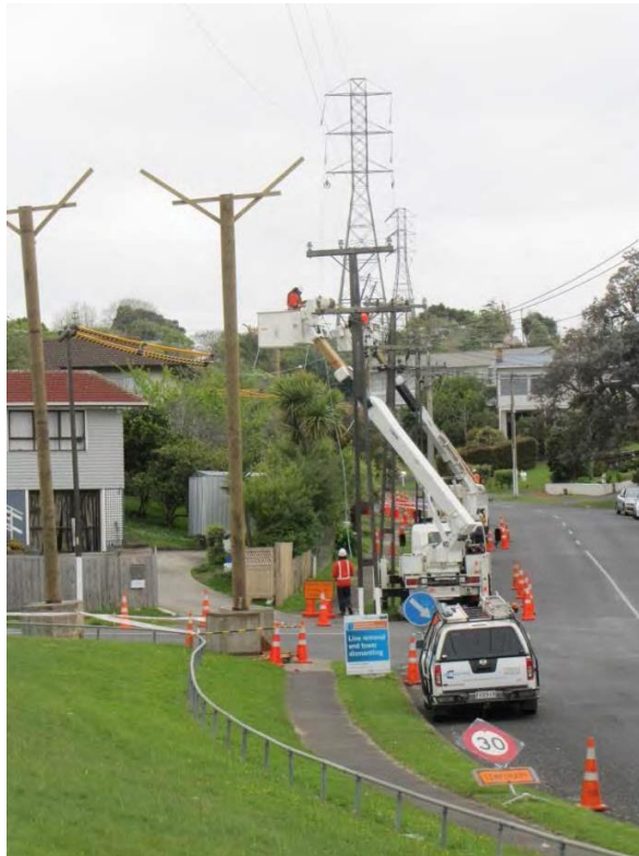
Figure 10: Removal of copper conductor on Pakuranga-Penrose A line, Auckland
