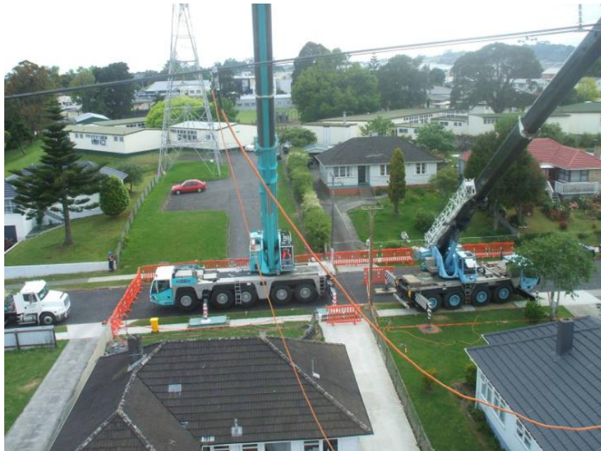
Figure 14: Reconductoring in an urban setting
