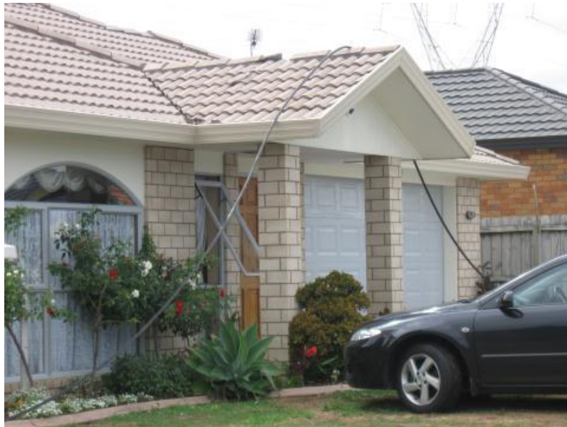
Figure 18: A conductor drop
