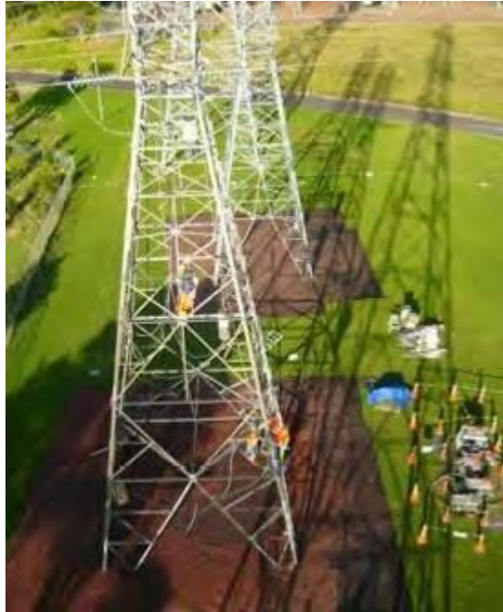
Figure 7: Abrasive blasting in area with no under-build — Auckland area
