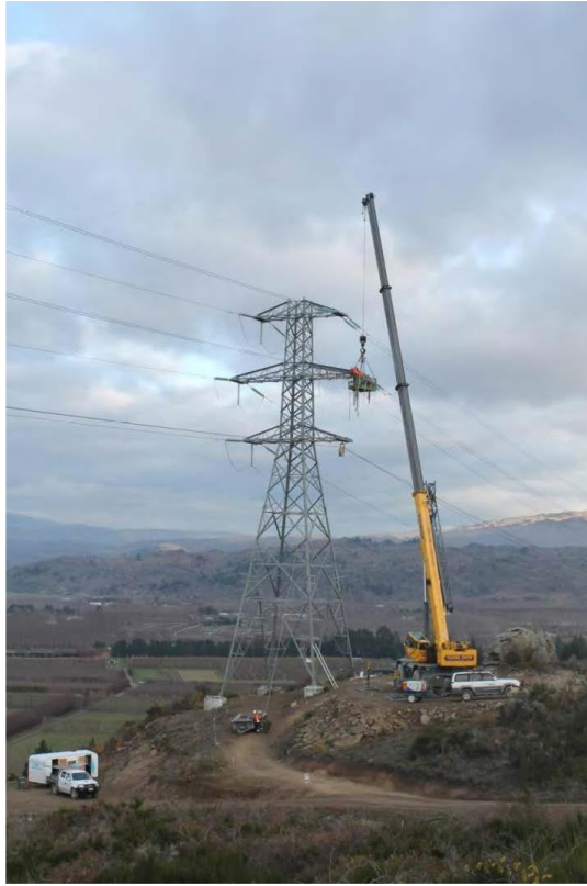
Figure 11: Crane being used for re-stringing – Central Otago
