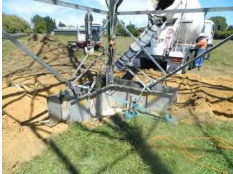
Figure 2: Grillage foundation replacement
