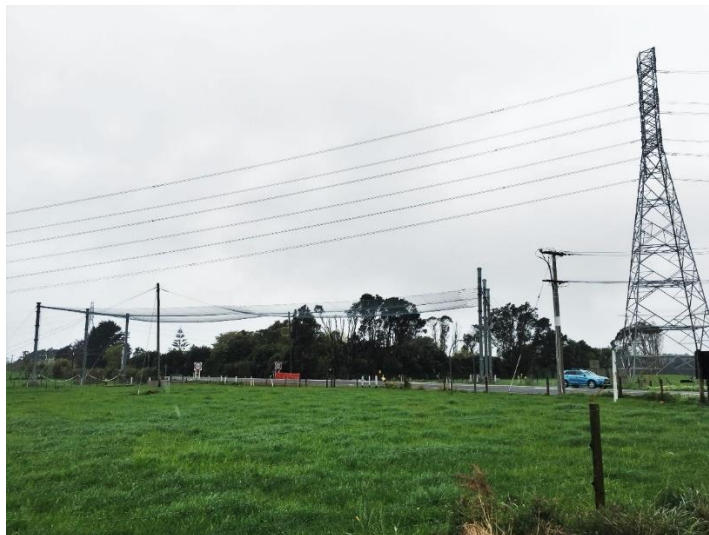
Figure 13: More substantial hurdles installed to mitigate potential conductor drop during wiring
