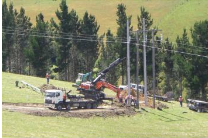
Figure 15: Pole replacement works, equipment and space required
