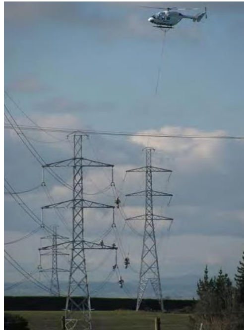
Figure 8: Maintenance work being carried out using helicopters
