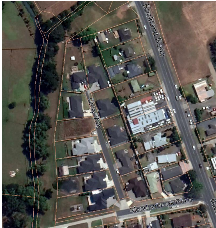
Figure 5: A 5.5m wide private carriageway provides two-way access to 10 allotments within a 10m wide reserve width
