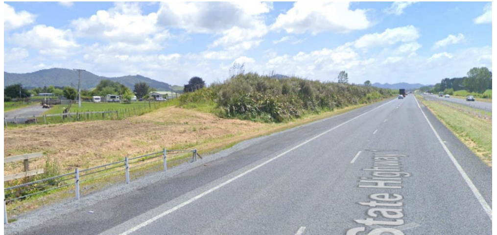
Drawing 2 - Earth works (bundling) approach – State Highway 1 Expressway section between Taupiri and Hamilton
