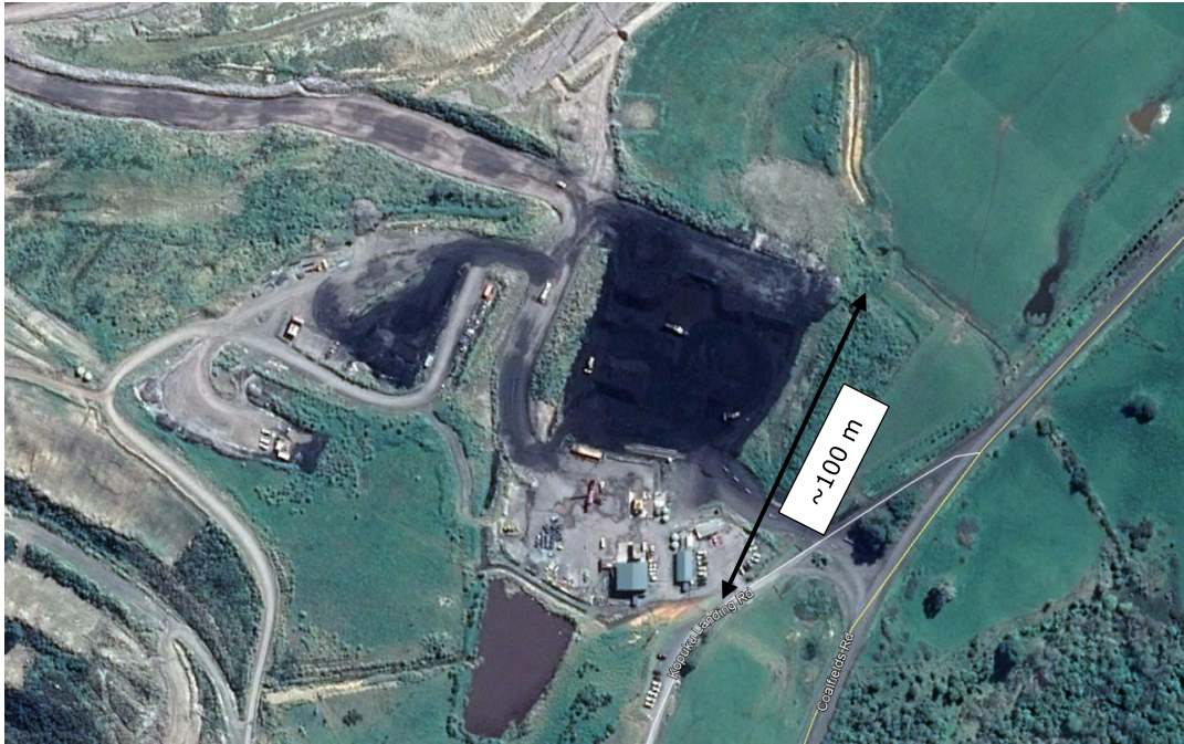
Figure 4 – Aerial Image of the Maramarua opencast infrastructure area
