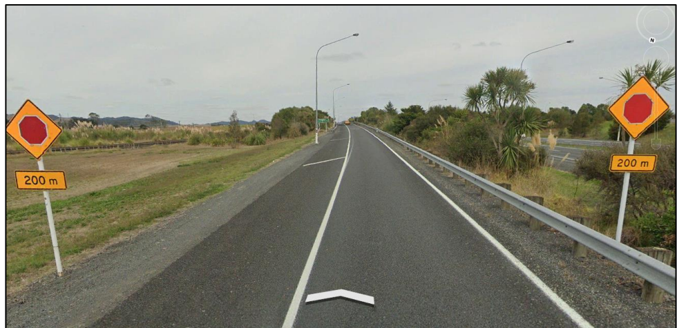
Figure 8: Southbound Off-Ramp at Ohinewai (Source: Google Street View)
