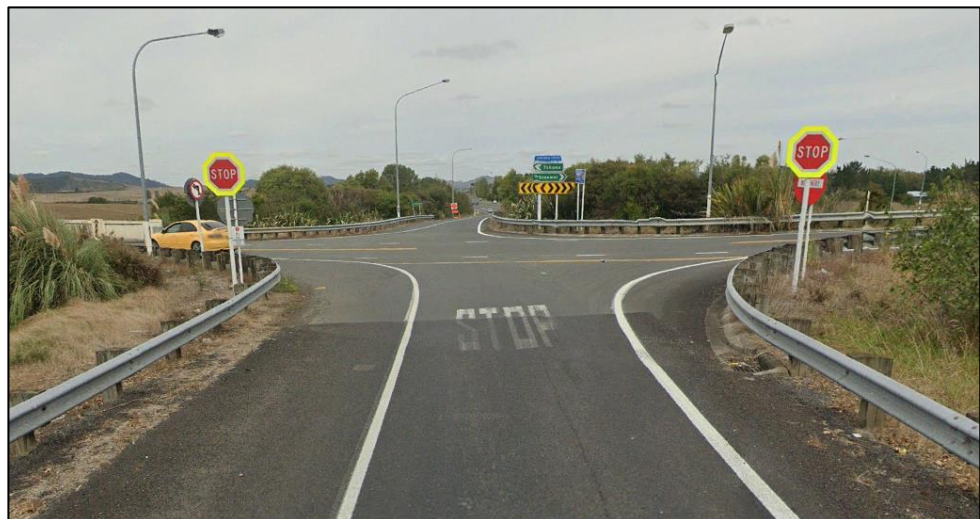
Figure 9: Southbound Off- Ramp intersection with Tahuna Road (Source: Google Street View)
