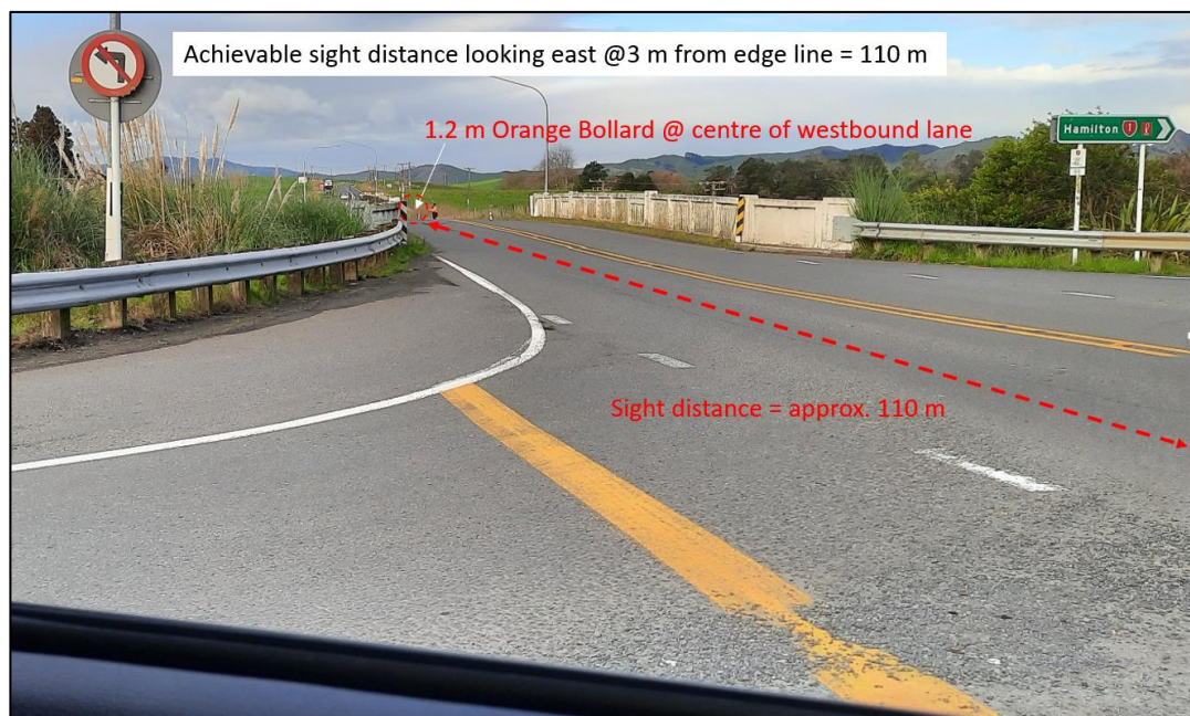
Figure 30: Achievable sightlines looking east at the Ohinewai Interchange southbound off-ramp (3 m from edge line)
