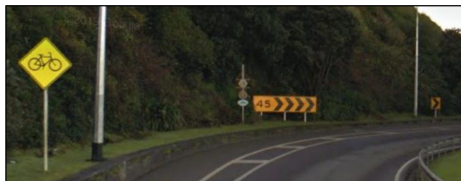
Figure 26: Static warning signs on the Petone northbound off-ramp, Wellington (Source: Google Street View)
