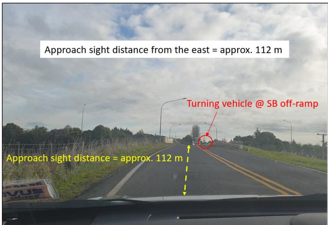
Figure 31: Approach sight distance from the east of the Ohinewai Interchange southbound off-ramp
