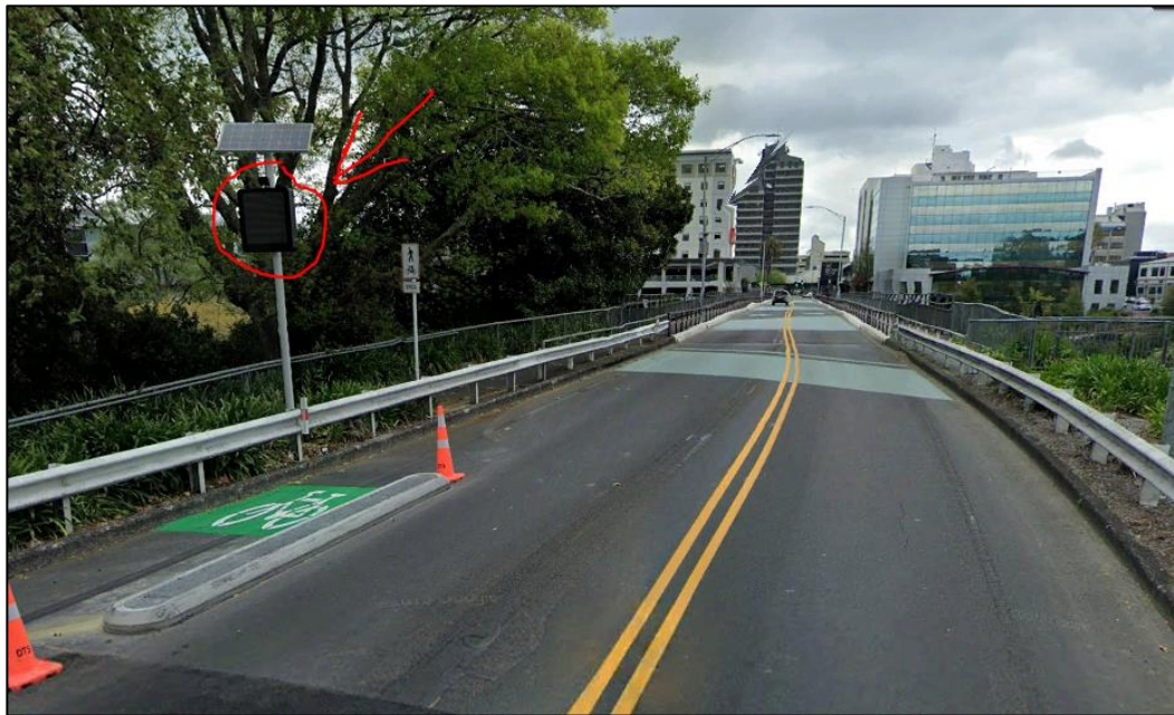
Figure 24: Electronic Messaging Signs at the Claudelands Bridge, Hamilton (Source: Google Street View)
