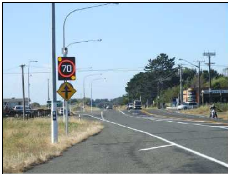
Figure 2: Rural Intersection Activated Warning Signs (RIAWS)
