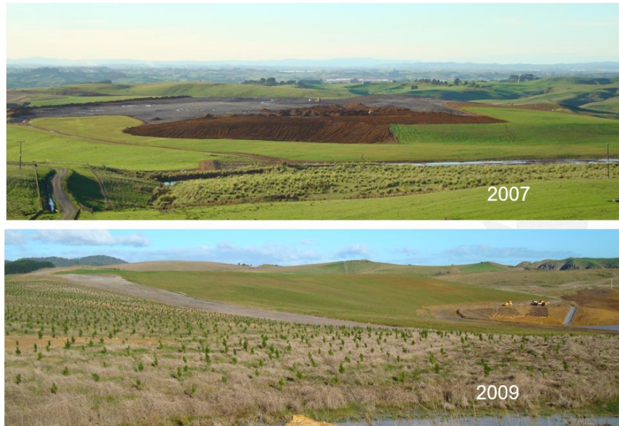
Figure 10: Recent rehabilitation at Rotowaro’s Township Opencast. The 2007 image shows rehab soils being spread along-side recently grassed slopes. The 2009 image shows similar rehabilitation process but the foreground surfaces have been planted in pine. A long-term drain (linear grey structure) is being constructed (right hand side) at the foot of the recently completed slope.
