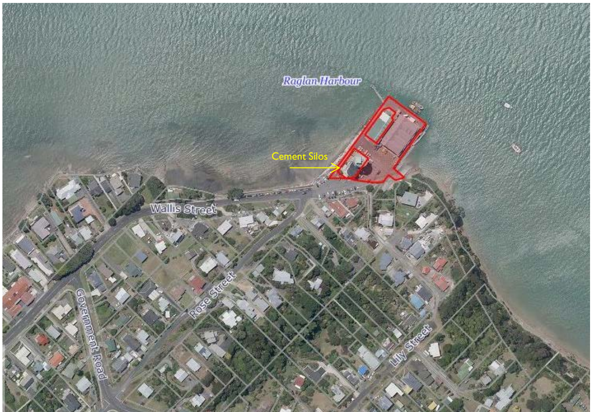
Figure 6: Raglan Wharf and location of the cement silos
