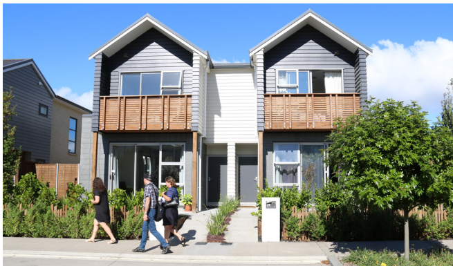
Figure 7. Precedent Image: Clearly visible front entrance.
