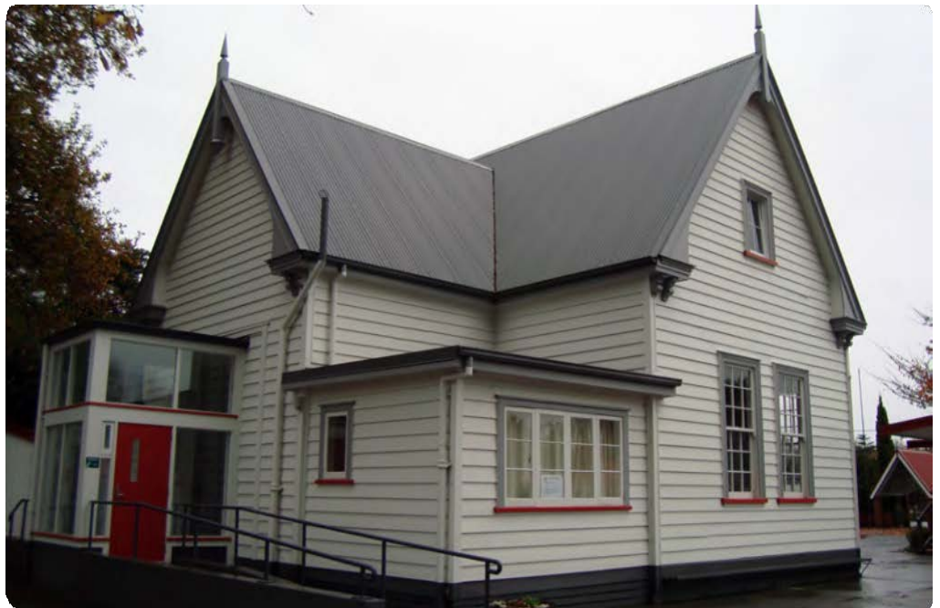
Figure 1. Tamahere School Original Building
