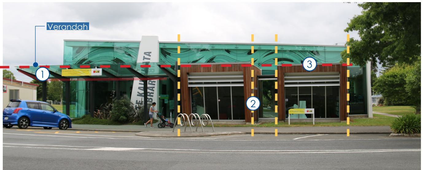
Figure 2. Te Kauwhata Library - a modern interpretation of existing built form, with verandah cover (1), vertical (2) and horizontal (3) modulation and a relatively flat roof form.
