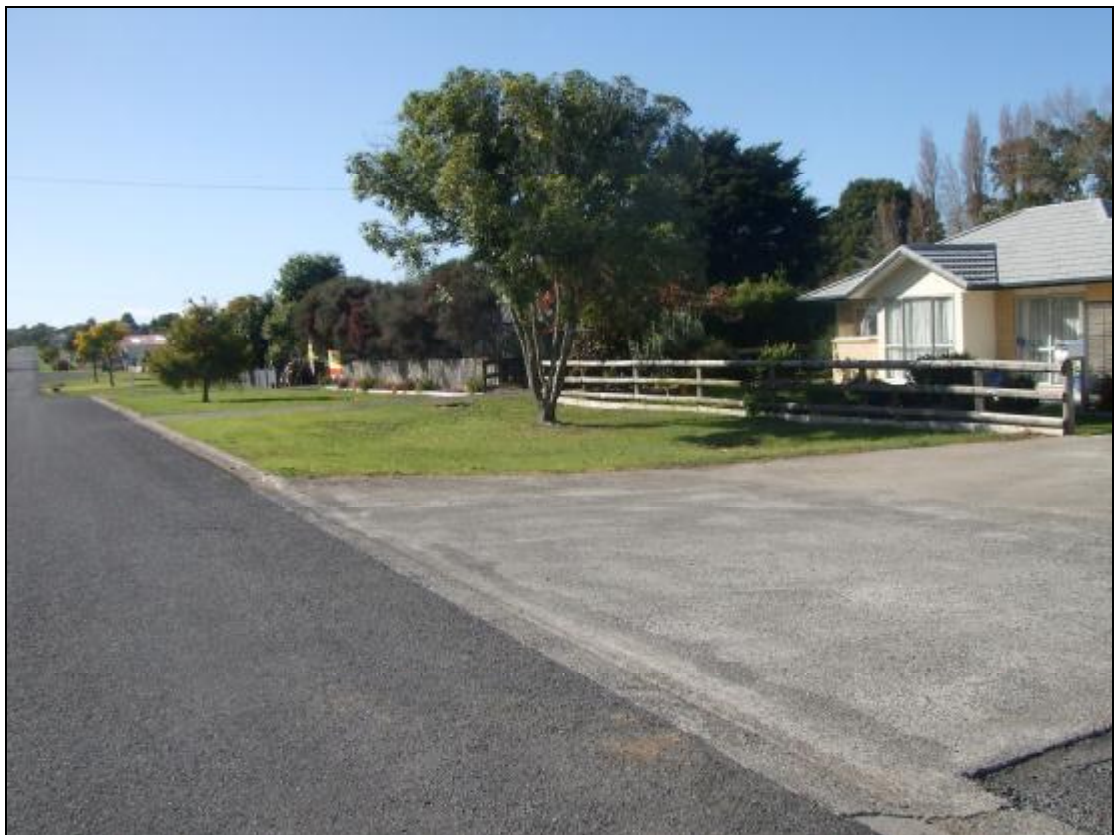
Photograph 6: The property located on the corner of Mahi Road and Saleyard Road; this property is regularly inundated
