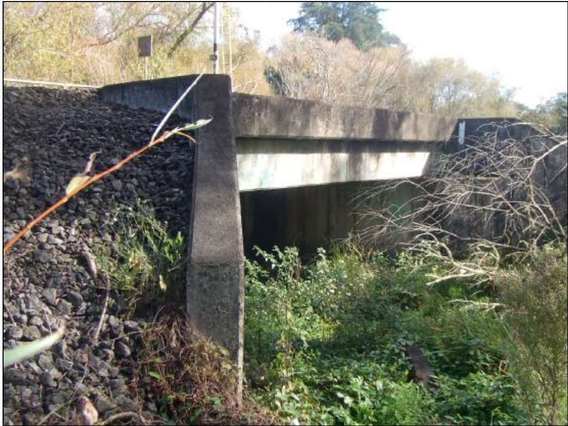
Photograph 7: The outlet of the railway bridge, Travers Road catchment
