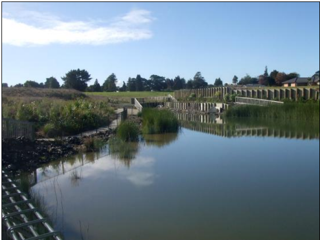
Photograph 4: The stormwater treatment pond located at the recent Blunt Road sub-division
