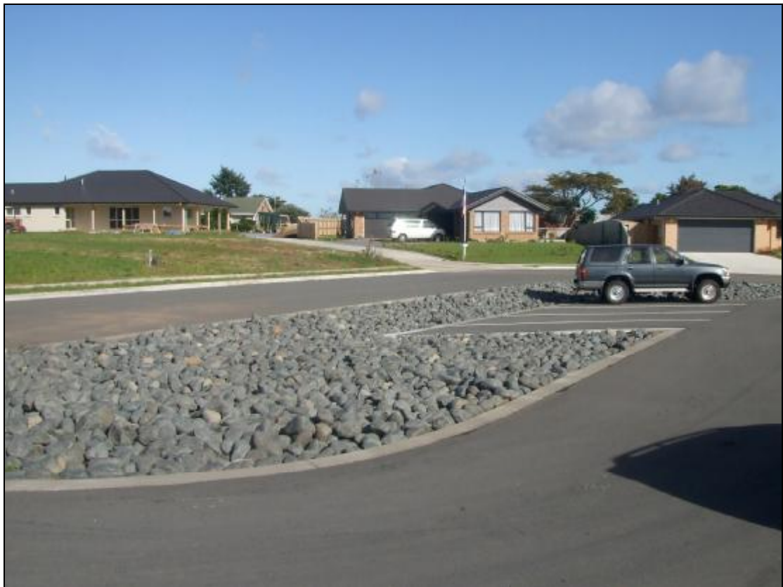
Photograph 2: Stormwater treatment device located on Roto Street
