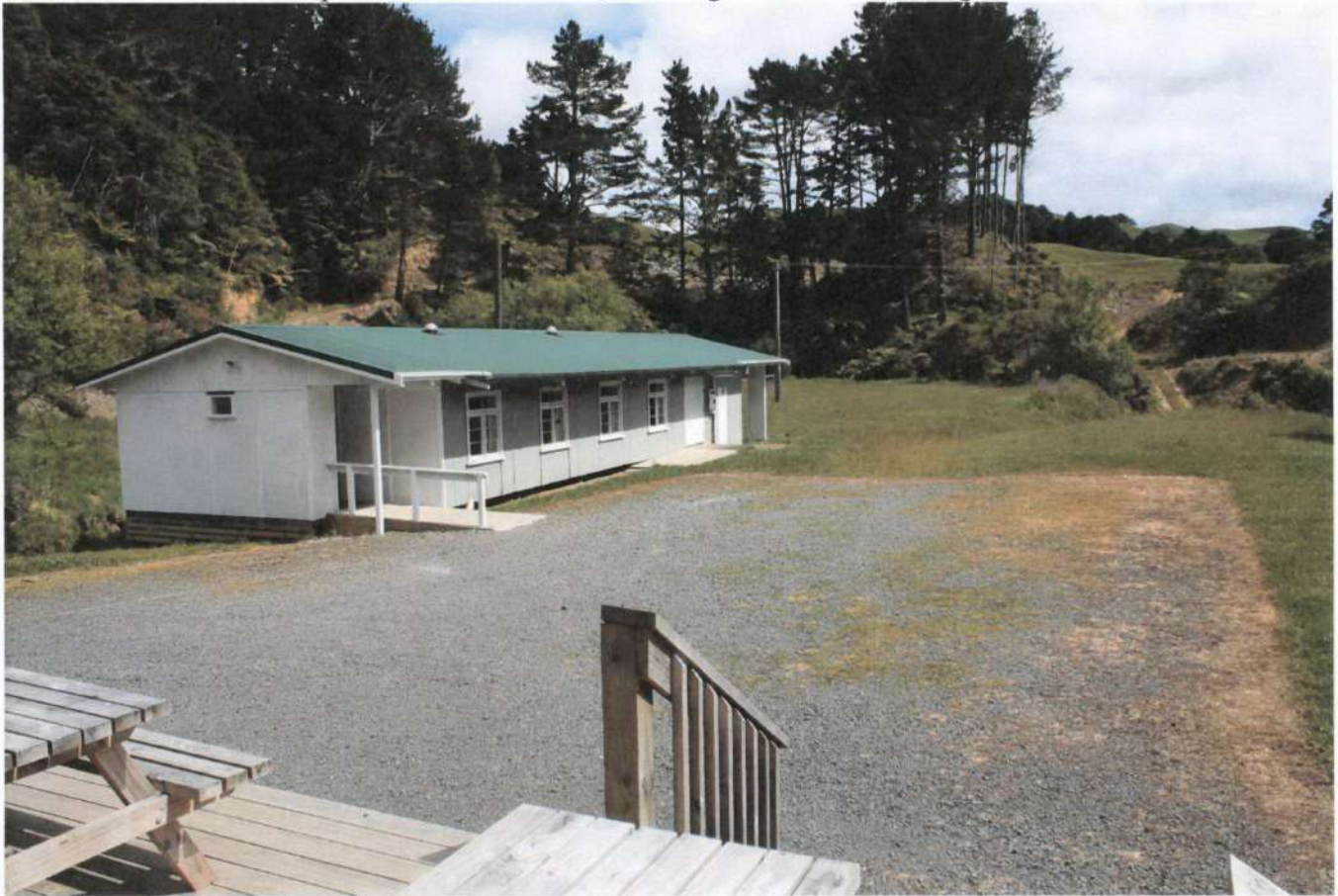
General view of the Camp from main hall deck, showing bunkroom building
