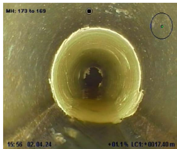
CCTV view after pipe repair
