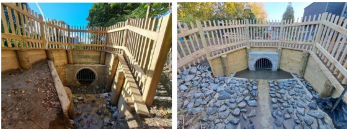
Cambrae Road Culvert Upgrade – Upstream and Downstream headwalls
