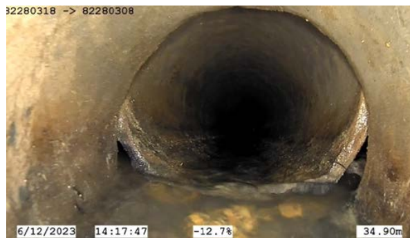
Cracked pipes
