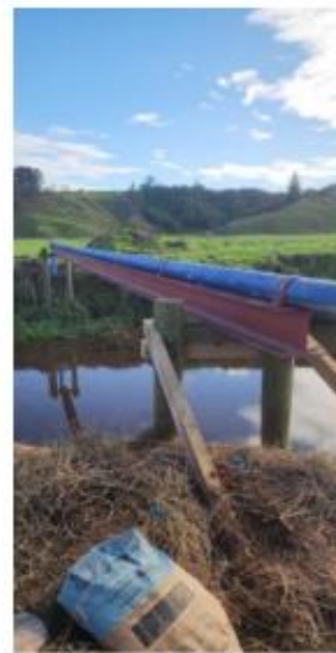
Replacement beam in place
