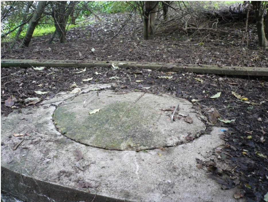
Figure 7 Western District Zone Reservoir Lid
