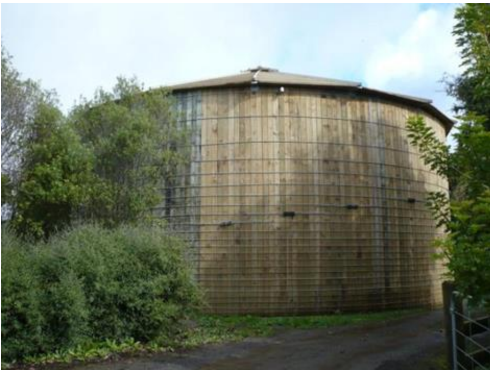
Figure 8 Harrisville Road Timber Reservoir
