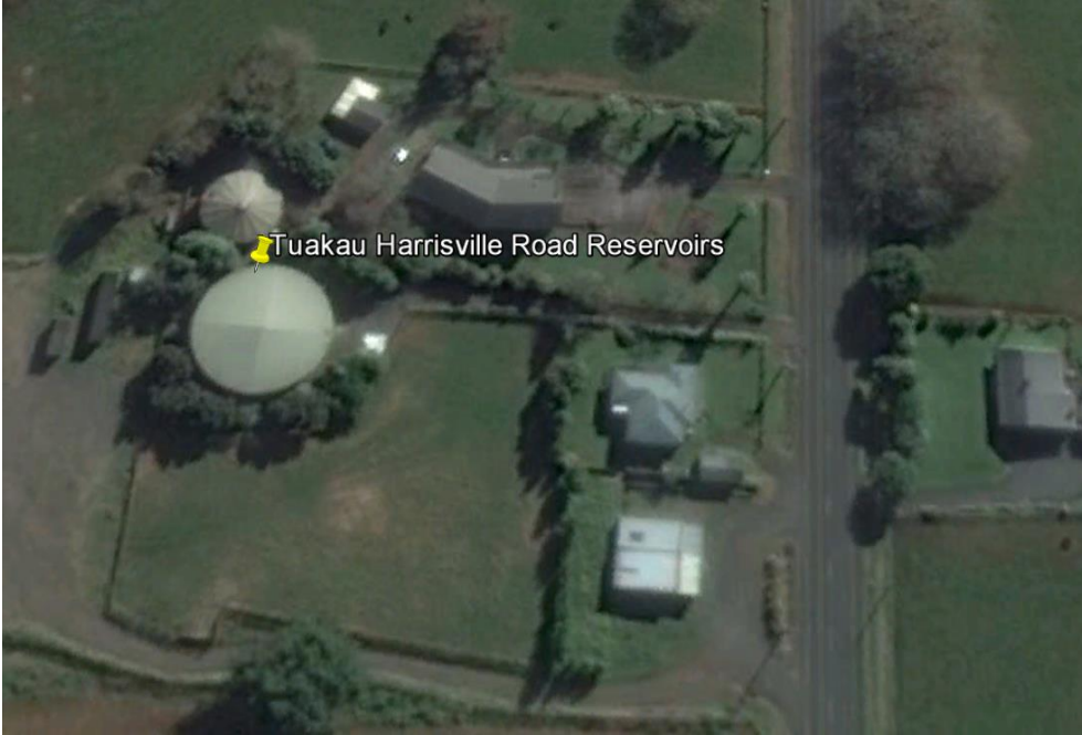
Figure 5 Harrisville Road Reservoirs
