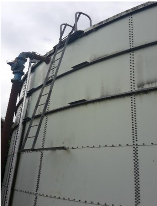
Figure 7 Harrisville Road Steel Reservoir – Ladder Detail
