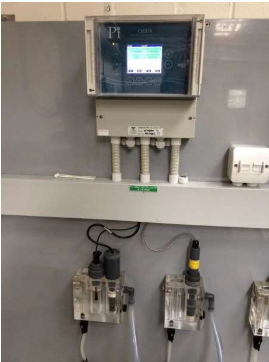
Figure 27. Filtered Water Quality Monitoring Instrumentation
