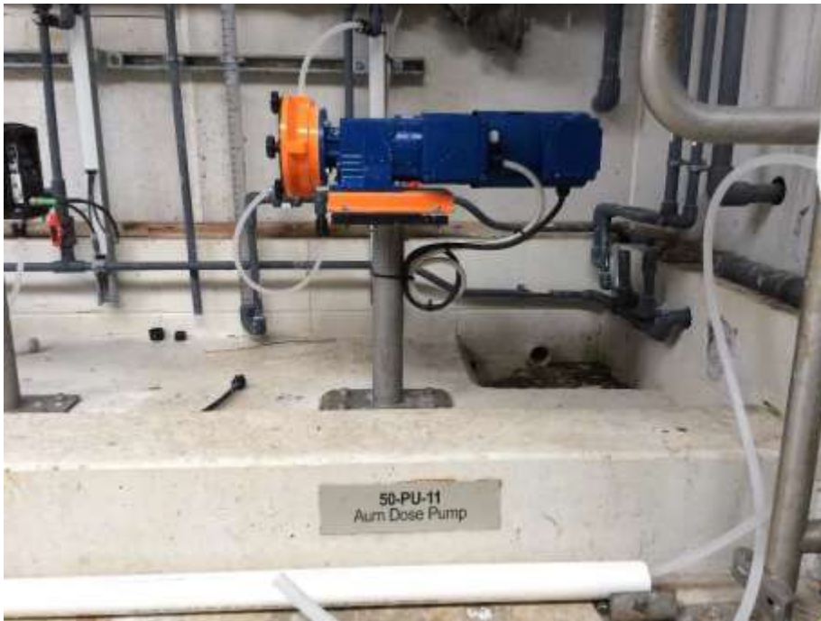
Figure 11. Alum Dosing Equipment
