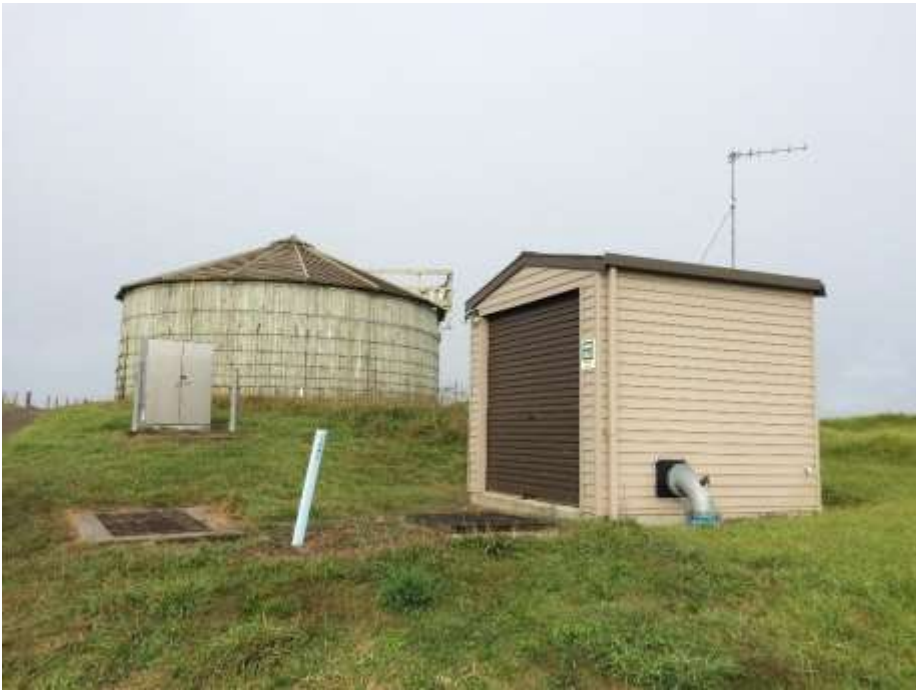
Figure 8 Raw Water Reservoir
