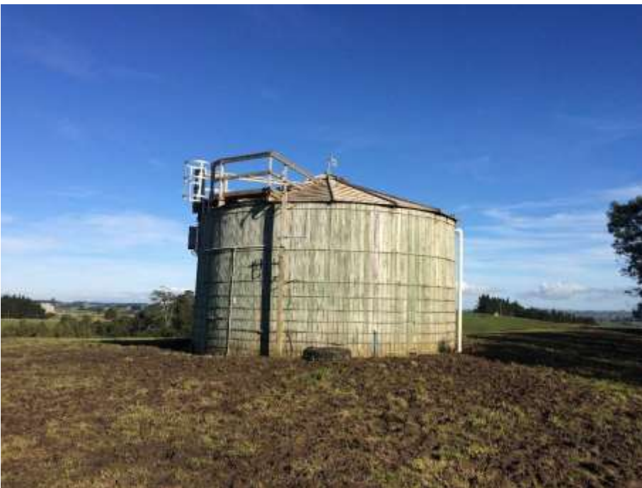
Figure 33. Network Reservoir, Springhill Road, Meremere
