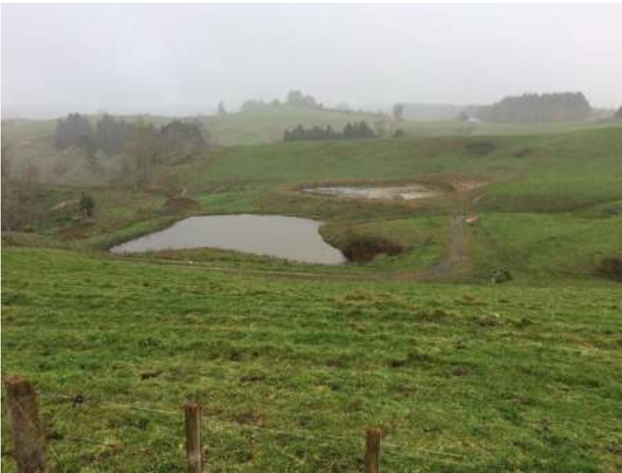
Figure 21. Clarifier and Filter Waste Settling Ponds
