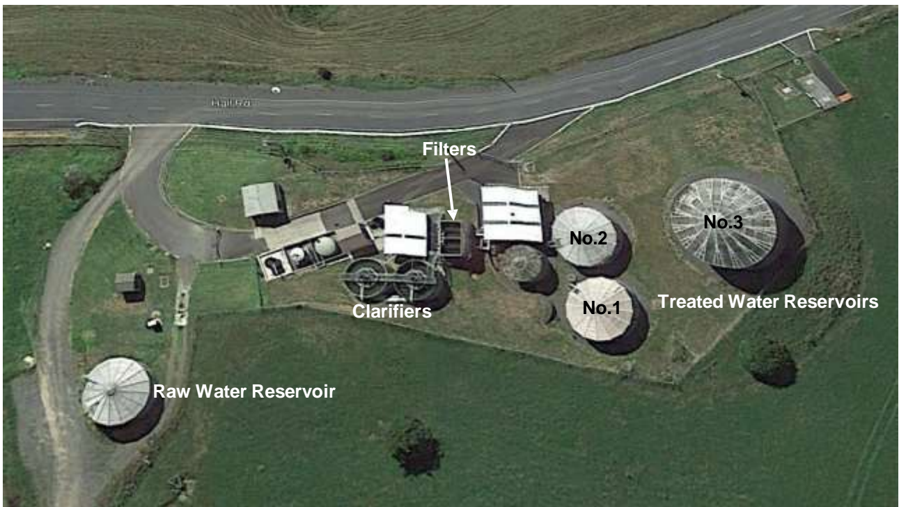
Figure 4. Te Kauwhata Treatment Plant Overview
