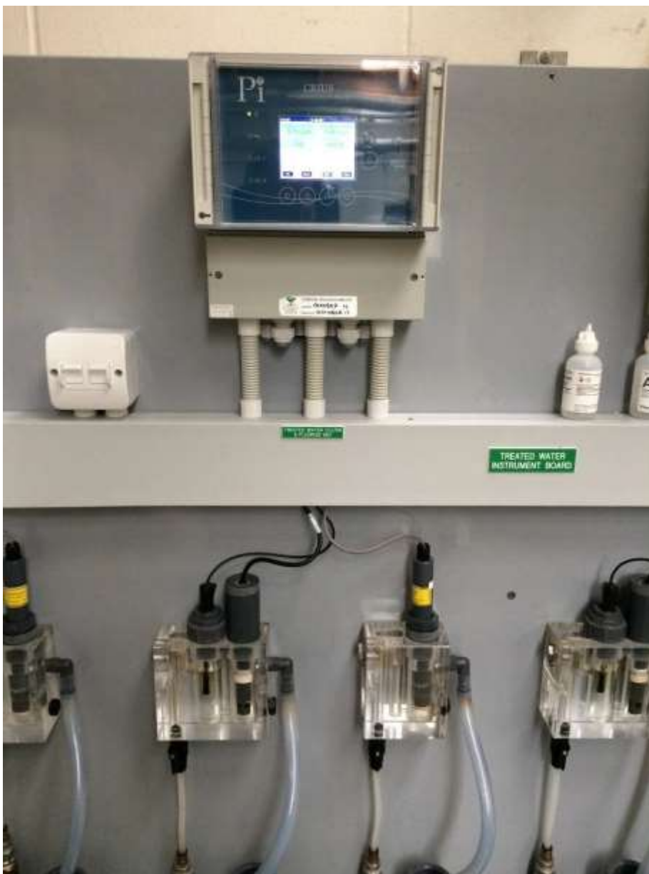
Figure 30. Final Water Quality Monitoring Instrumentation 1
