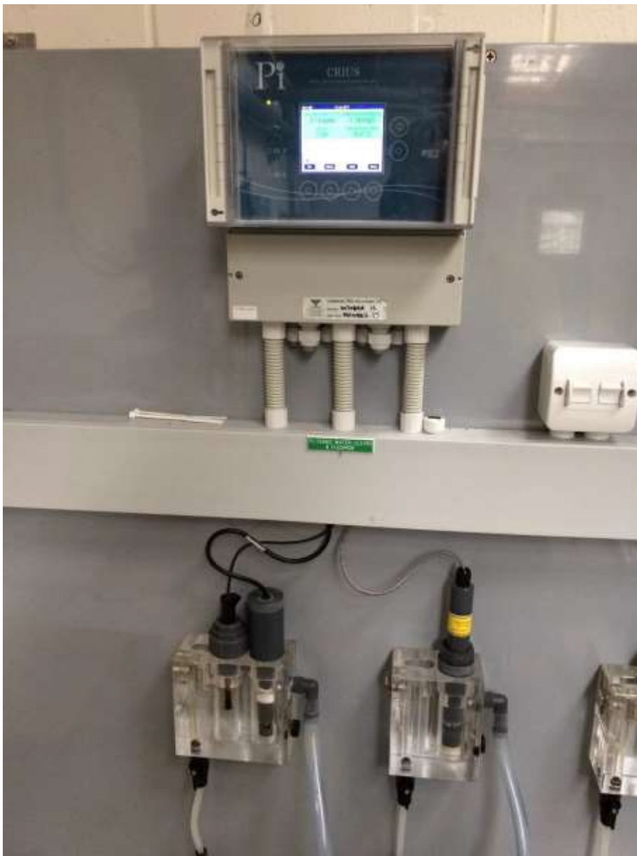
Figure 20. Filter Turbidimeters
