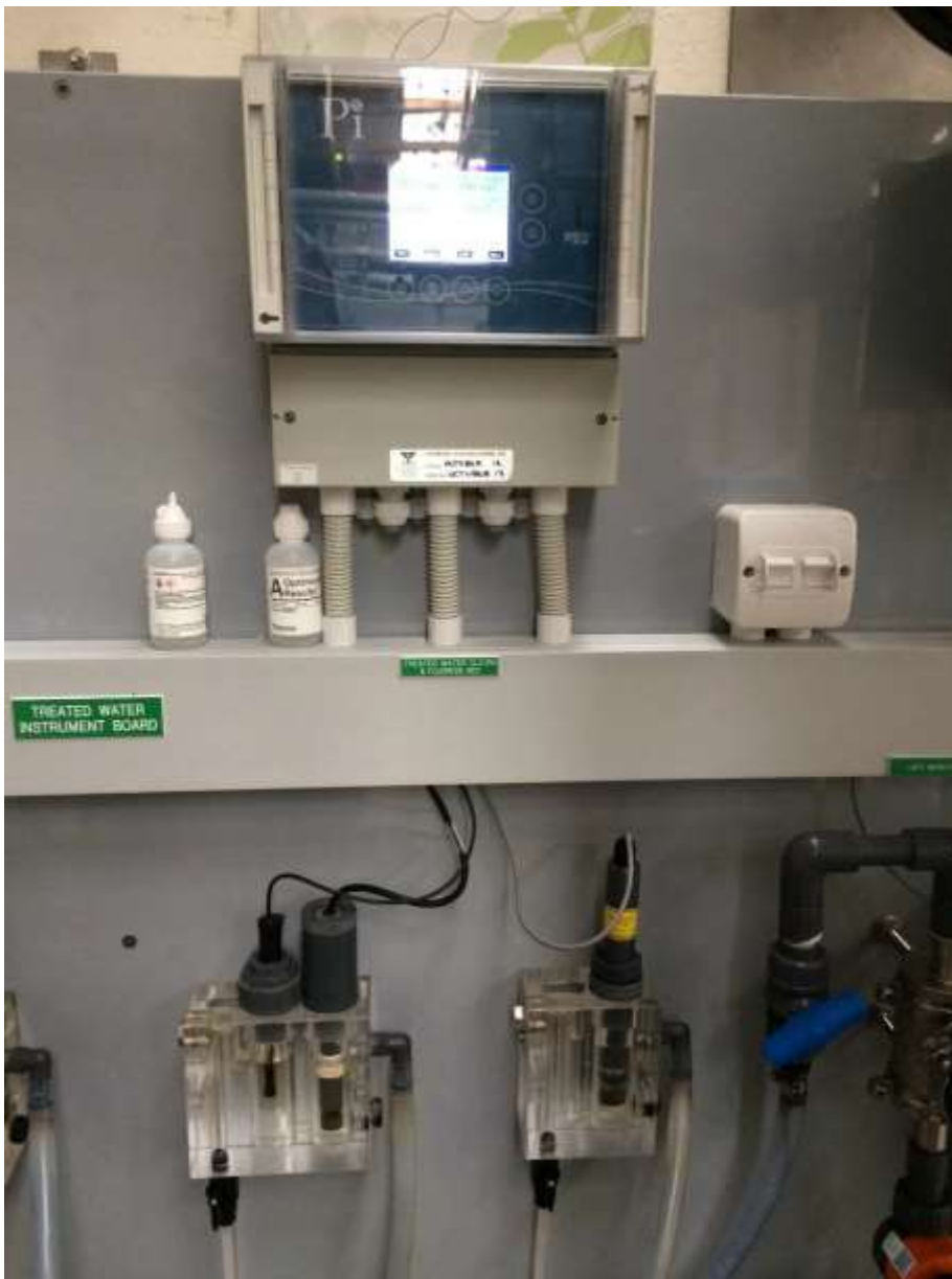
Figure 31. Final Water Quality Monitoring Instrumentation 2
