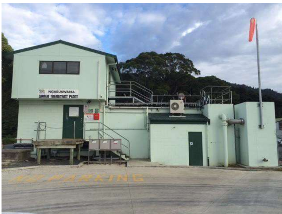
Figure 3 Water Treatment Plant – Lower Section
