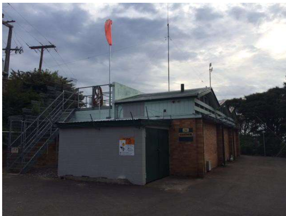
Figure 8. Water Treatment Plant – Upper Section
