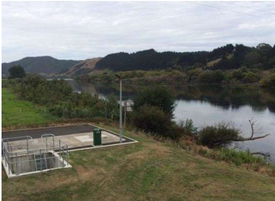
Figure 2 Intake and Raw Water Pumps Wet Well
