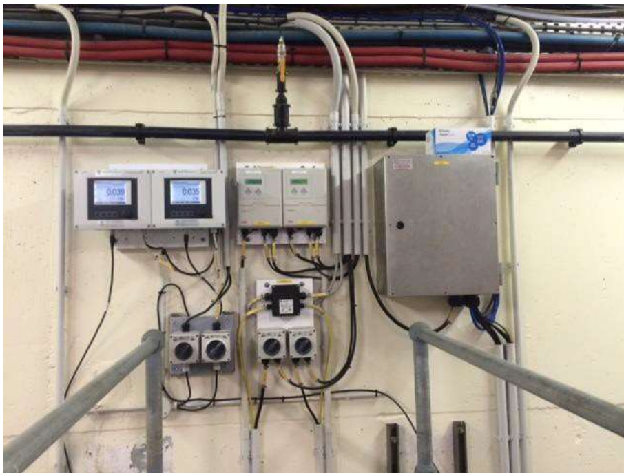
Figure 9. 2 of the 5 Filter Turbidimeters
