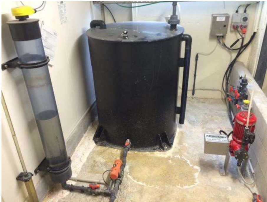
Figure 11. Alum Dosing Equipment
