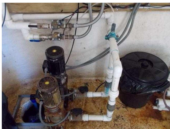
Figure 3. Spring abstraction and pumps
