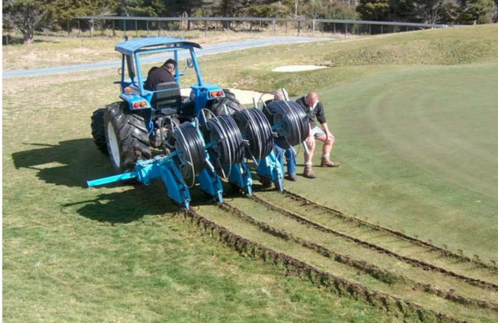
Figure 4: Top: Subsurface Drip Irrigation beneath Pasture 4 Btm: subsurface drip beneath a golf course 5
