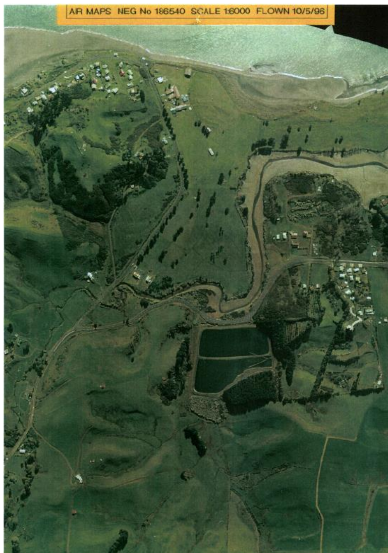
Figure 1.2: Raglan Wastewater Treatment Plant Oxidation Ponds as at May 1996 2
