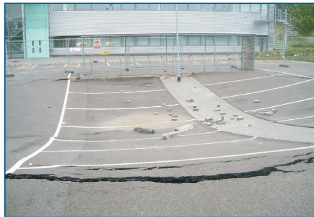
Example of the consequences of failure of a modular geocellular tank after three years
