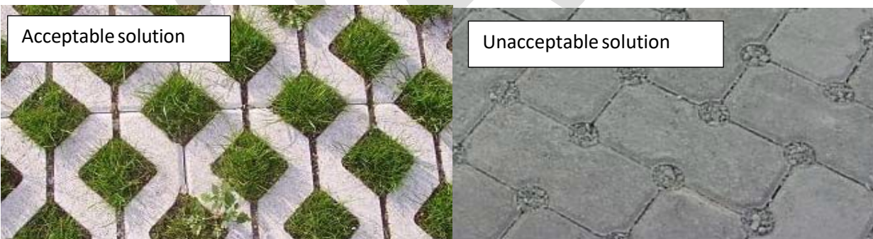
Figure 1: PerVIOUS pavement acceptable and unacceptable options
