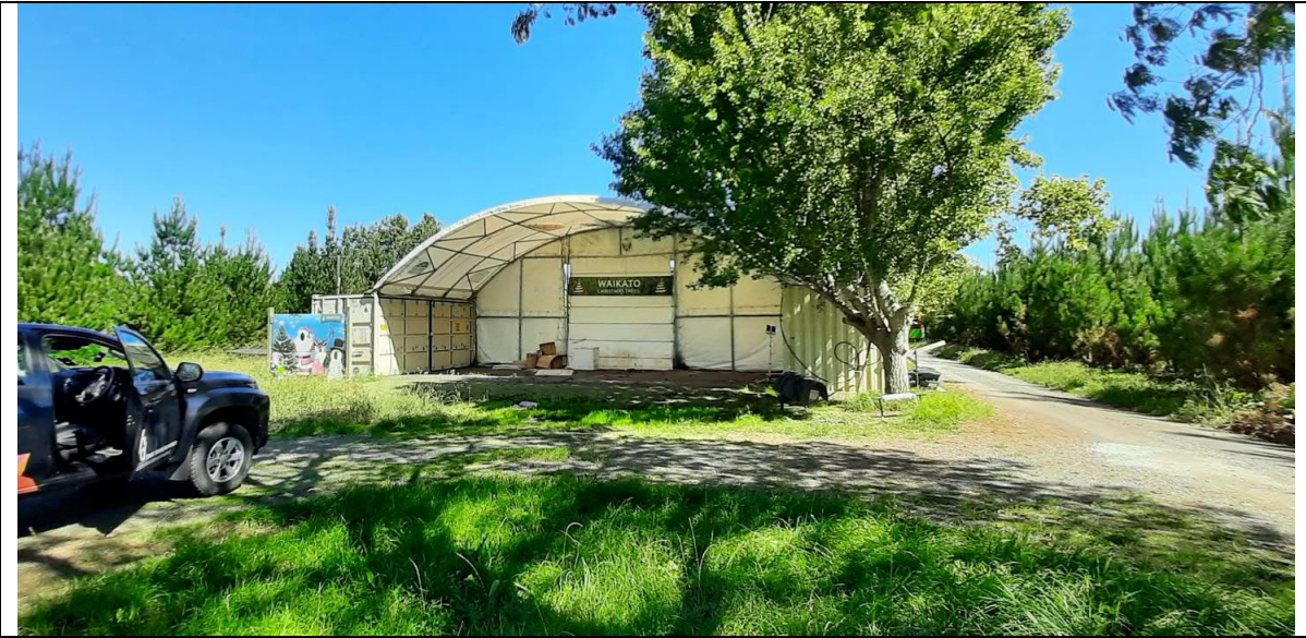
Photo 10: Existing shelter at 92 Tamahere Drive, facing west
