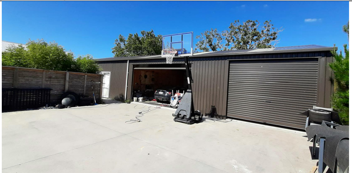
Photo 14: Existing shed at 92 Tamahere Drive, facing south
