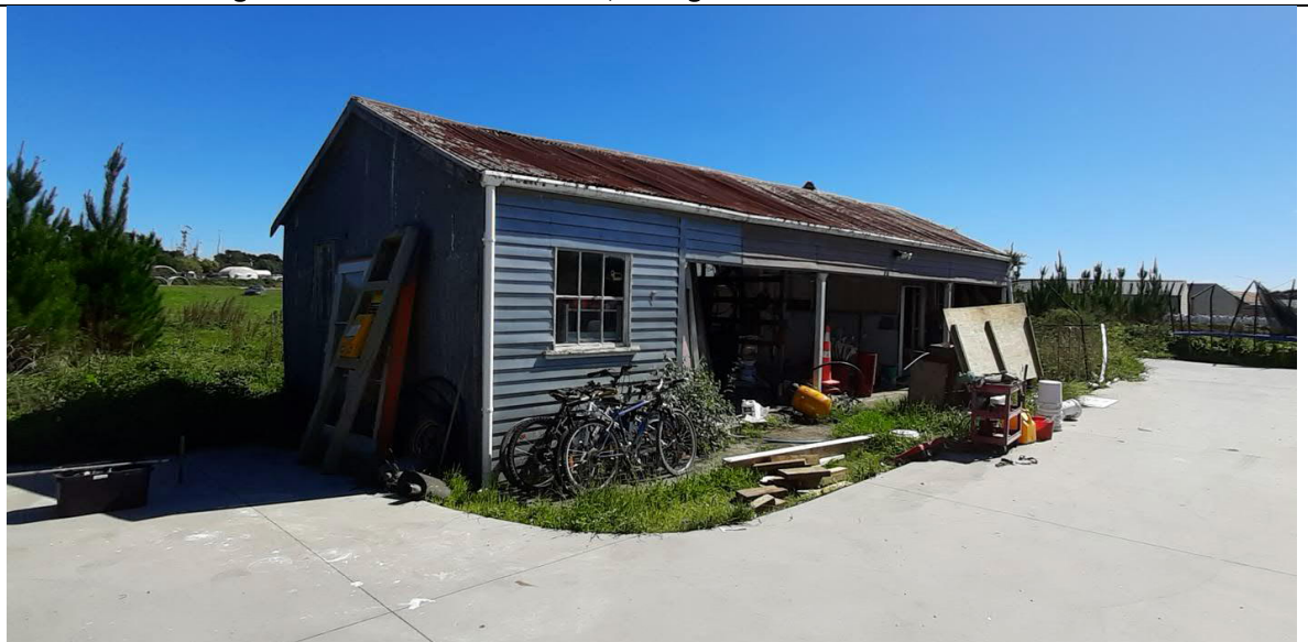
Photo 15: Existing shed at 92 Tamahere Drive, facing west
