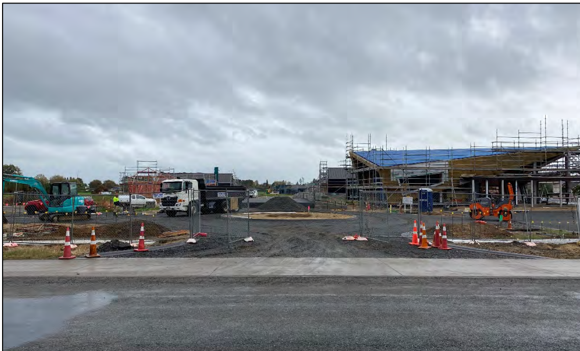
Figure 8: Tamahere Drive, Southern Access (Under Construction)
