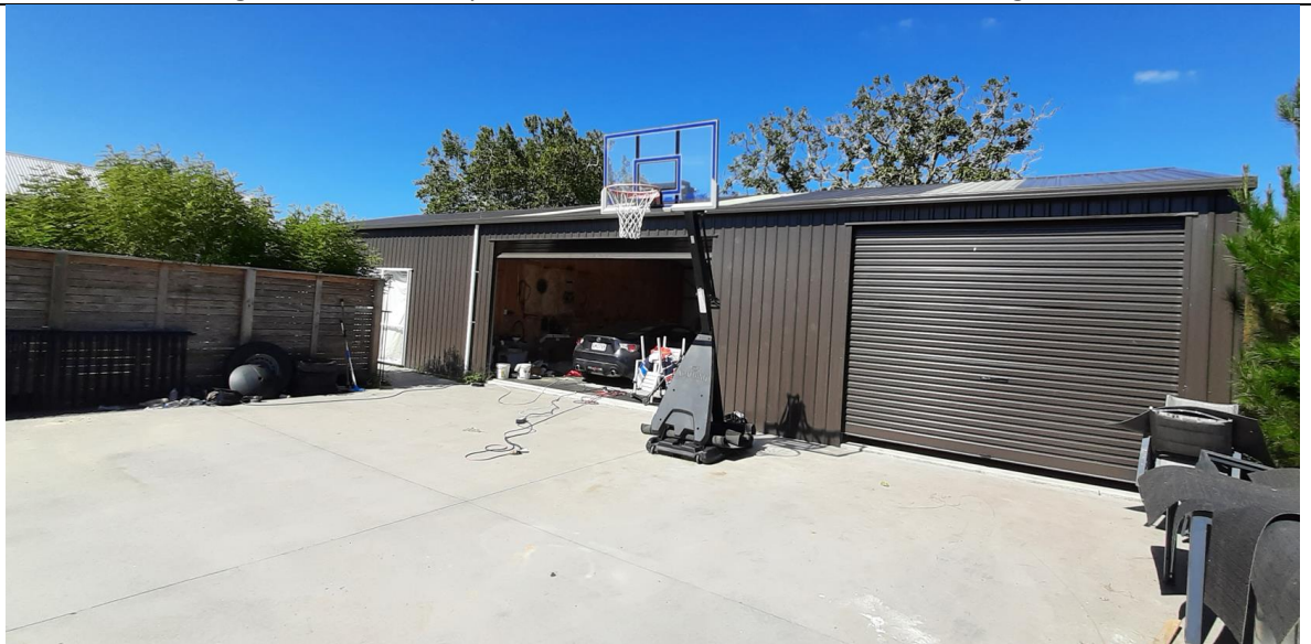
Photo 14: Existing shed at 92 Tamahere Drive, facing south
