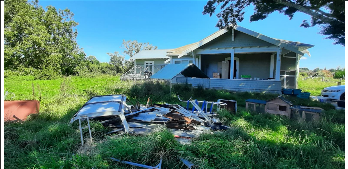
Photo 13: Existing house and stockpiled rubbish at 92 Tamahere Drive, facing west
