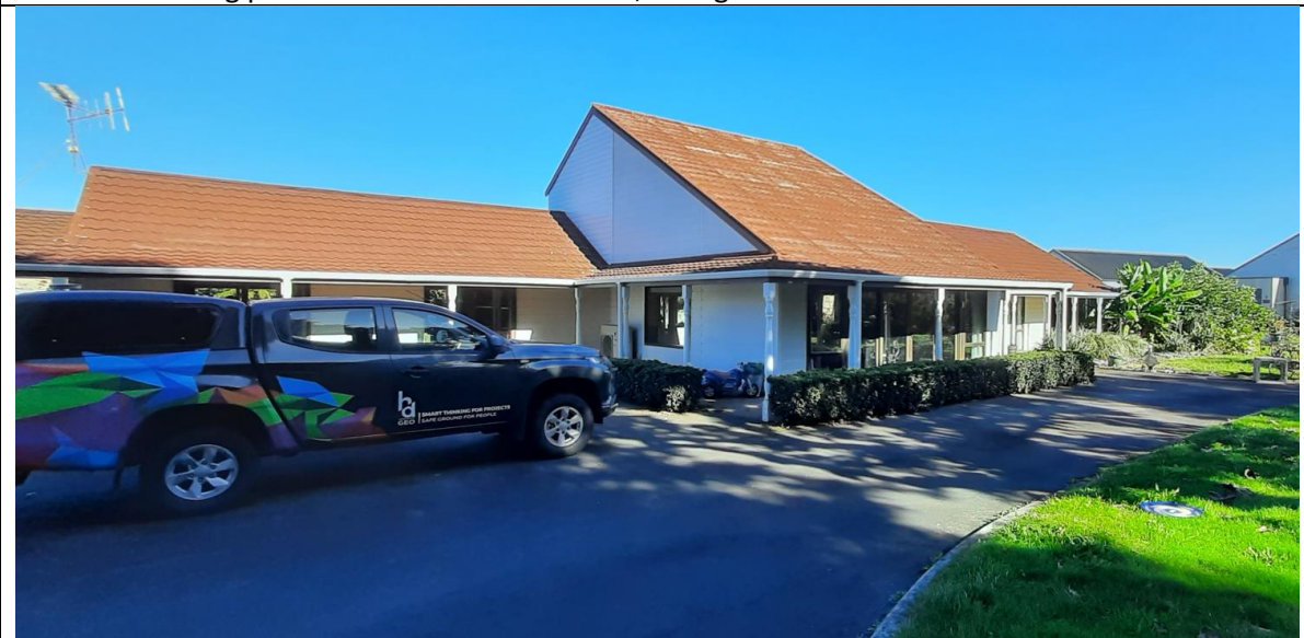
Photo 3: Existing house at 56 Tamahere Drive, facing south
