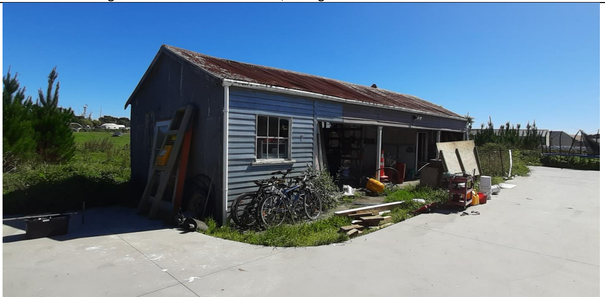
Photo 15: Existing shed at 92 Tamahere Drive, facing west
