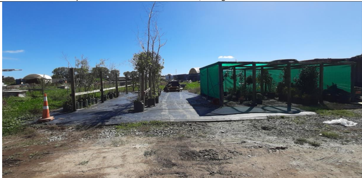
Photo 18: Recent laydown area at 92 Tamahere Drive, facing north
