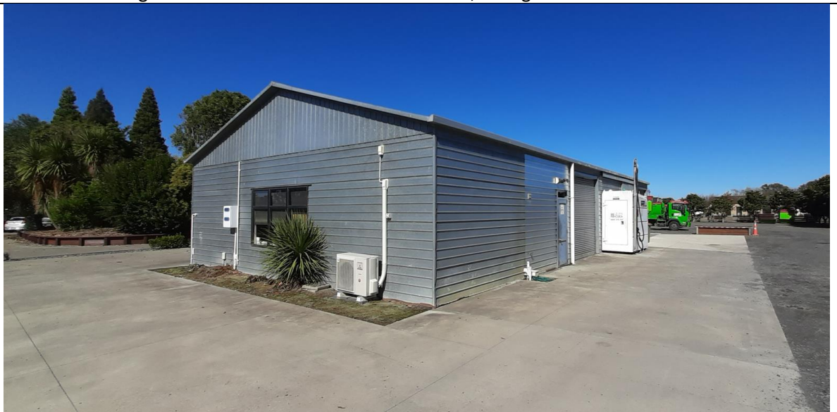
Photo 6: Existing commercial building (Red Lid) at 70 Tamahere Drive, facing west
