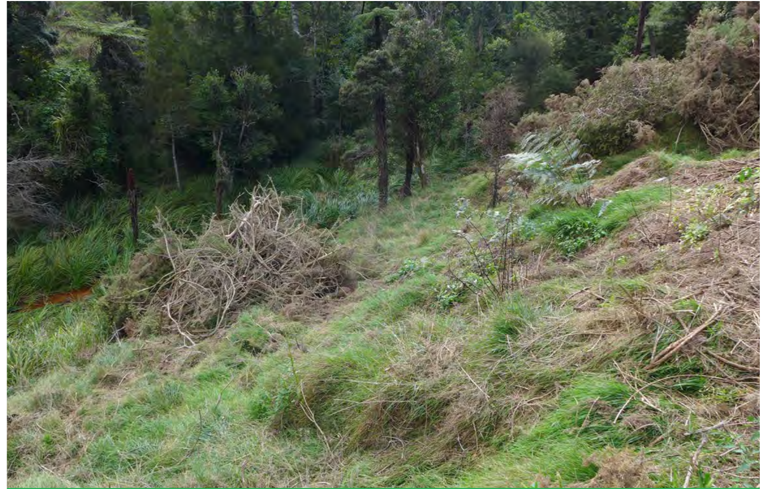
Figure 13: Gorse removed with chainsaws on the eastern side of the stream to prepare the area for planting.
