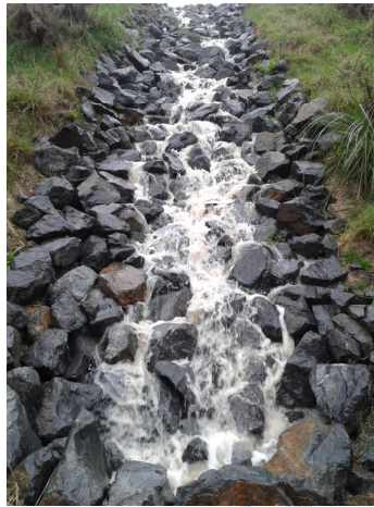
Photo 1 – Typical Quarry Rock Flume
