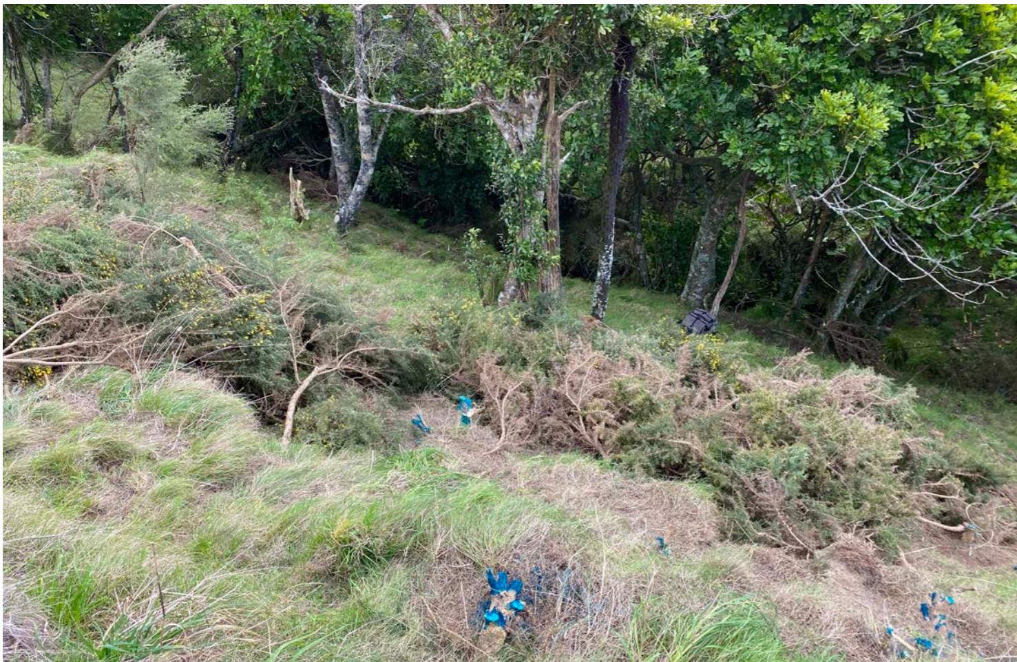
Figure 14: Gorse removed with a hand saw and grazon herbicide applied to cut stumps.
