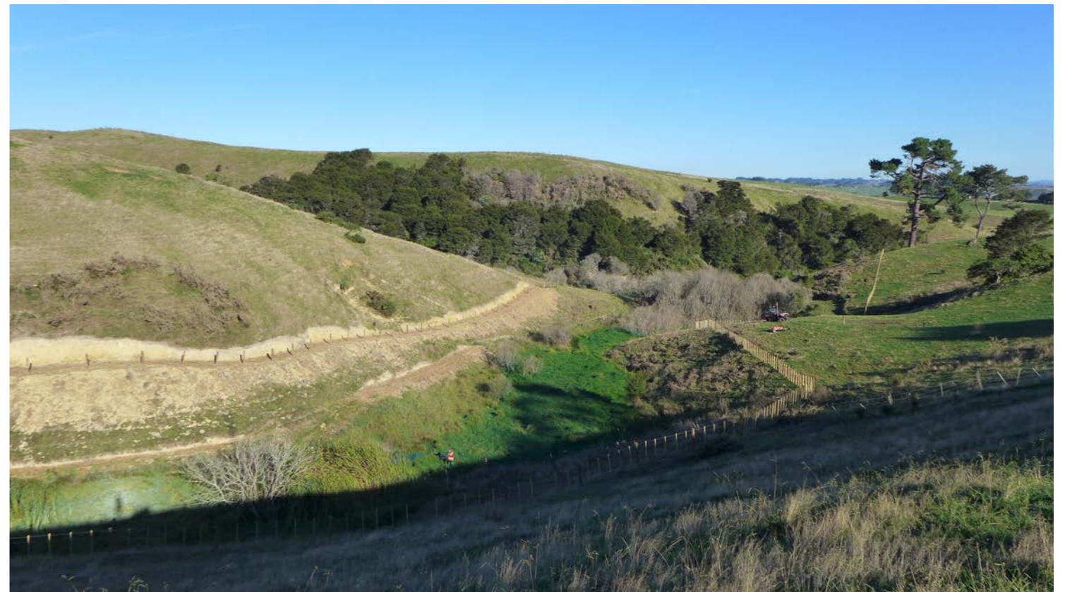
Figure 20: Fencing progress around the wetland, looking north-west. March 2022.
