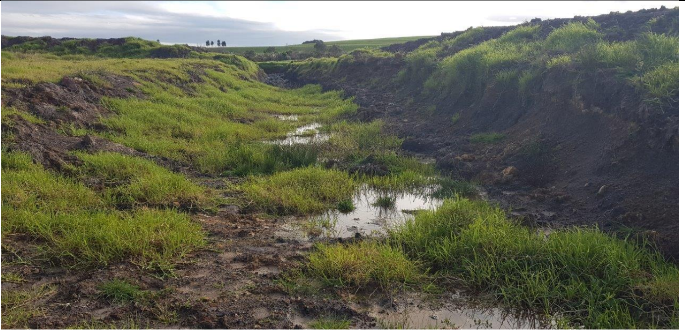
Figure 6: Outlet of pond area which appears to be at similar level to previous standing water level. Exposed areas to be seeded and mulched, or hydroseeded.
