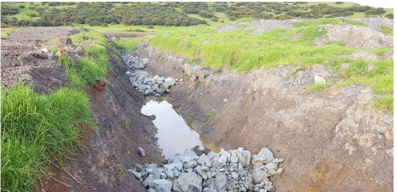
Figure 3: Check dams in southern branch of channel. Channel sides to be hydroseeded.
