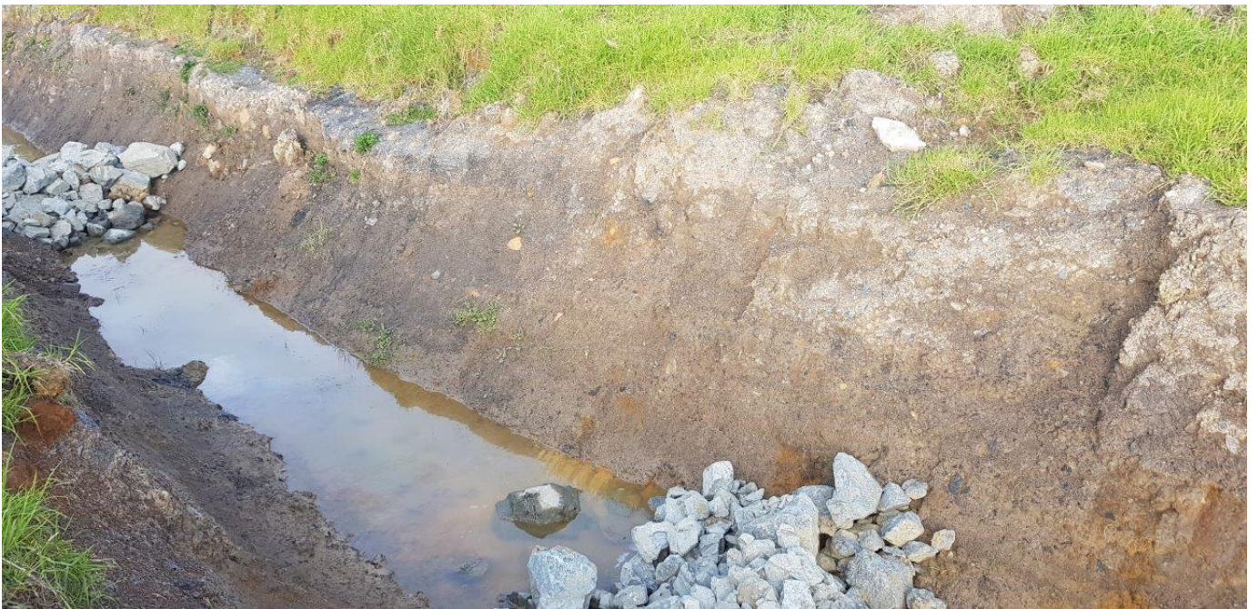
Figure 9: Existing channel sides and standing water. Channel sides to be hydroseeded.
