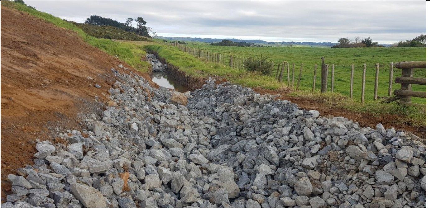
Figure 2: Upstream extent of outlet spillway and check dams in background. Channel sides to be hydroseeded and slope to left to be seeded and mulched.
