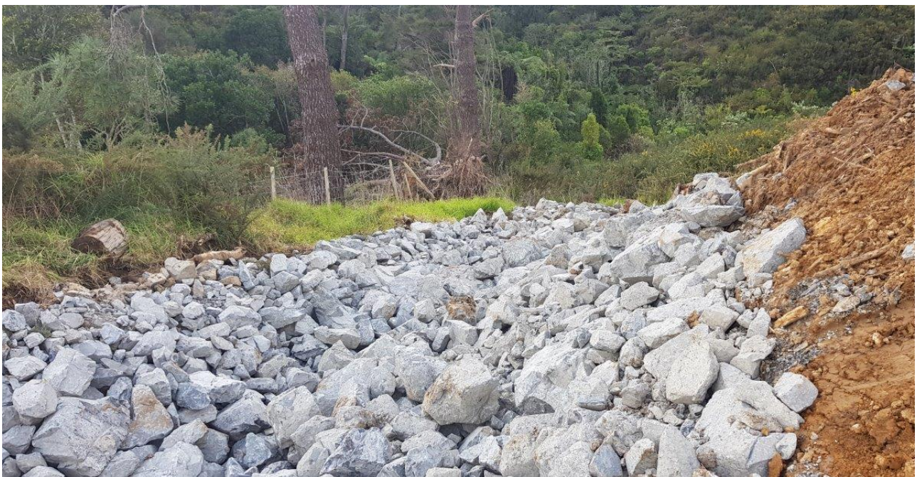
Figure 1: Outlet spill way. Slope to right to be seeded and mulched.
