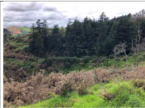
Plate 4-12: Dam face from across the valley
