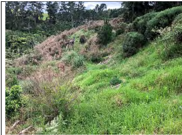
Plate 4-11: Top portion of the dam face
