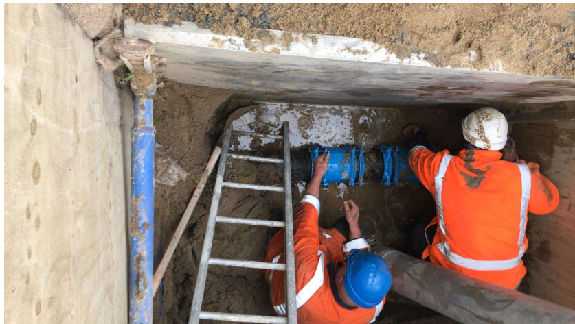
Repair being completed – new Gibault installed.
