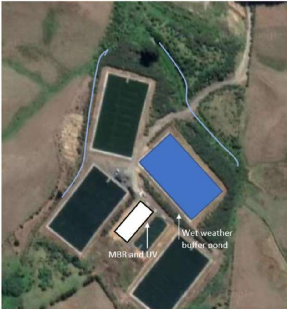
Image: Theoretical layout of a Raglan MBR plant (tributaries leading to the upper harbour are indicated with blue lines. These would be the discharge locations)
