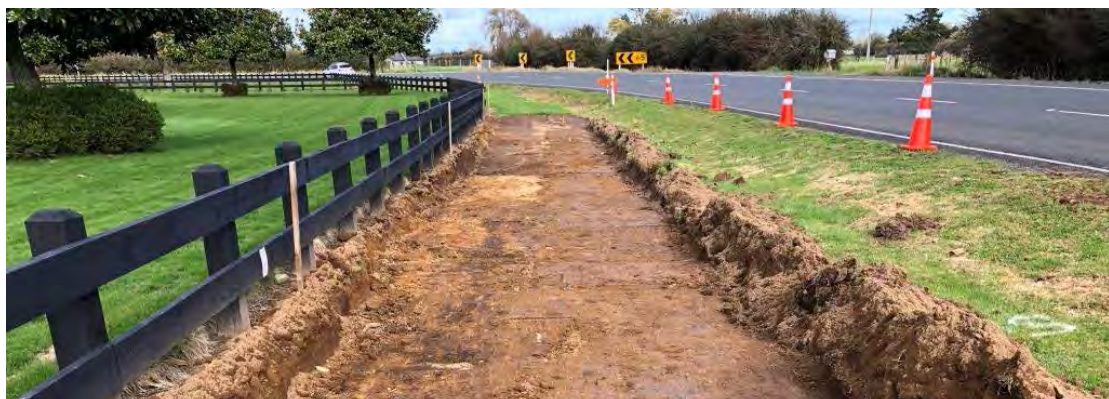
Newell Road Shared Path – Excavation underway 7/06/2018
