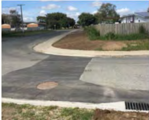
Reinstated looking towards Kent St and George St
