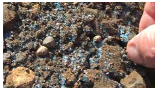
Blue Polycom granules applied to Phillips Road (Before blending into pavement)
