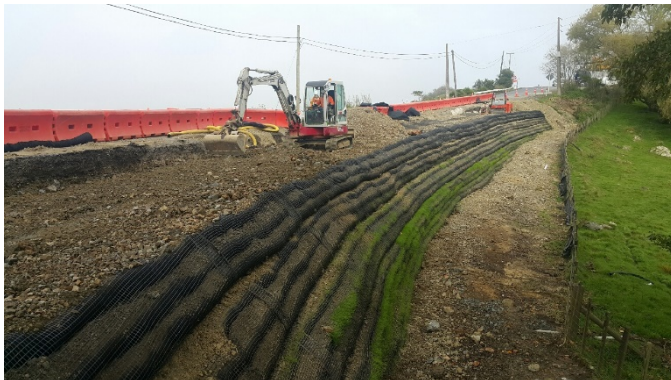
Highway 22 MSE Wall
