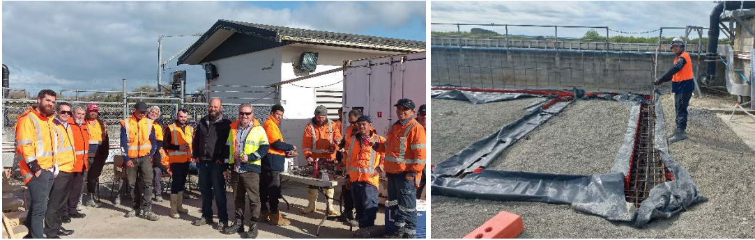
Te Kauwhata WWTP Upgrade: Commencement briefing and blower room foundation works
