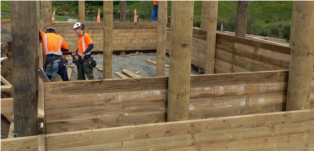
POAL WWPS – Barkbed Installation is underway
