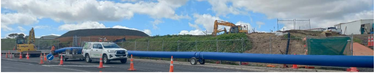
New reservoir town supply pipeline being pulled on
