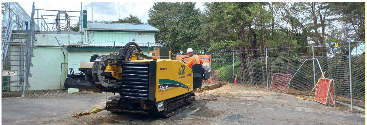
Ngaruawahia WTP Upgrade – Run to waste horizontal directional drill installation
