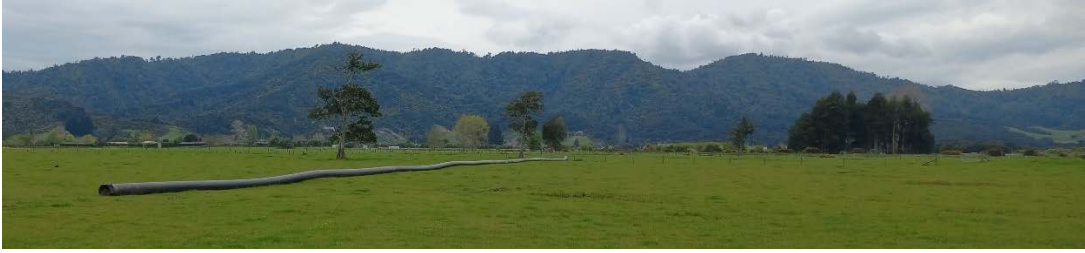
Ngāruawāhia Pipeline – Bypass Pipeline
