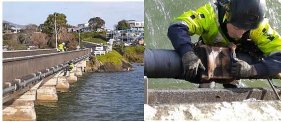
Abseilers carrying out gibbalt repair work
