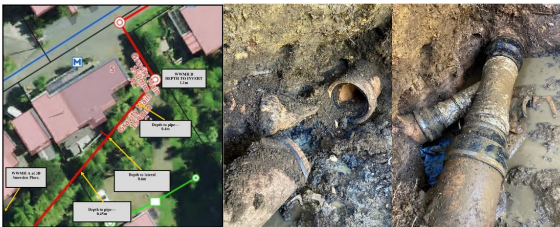
Before and after images of the line repair
