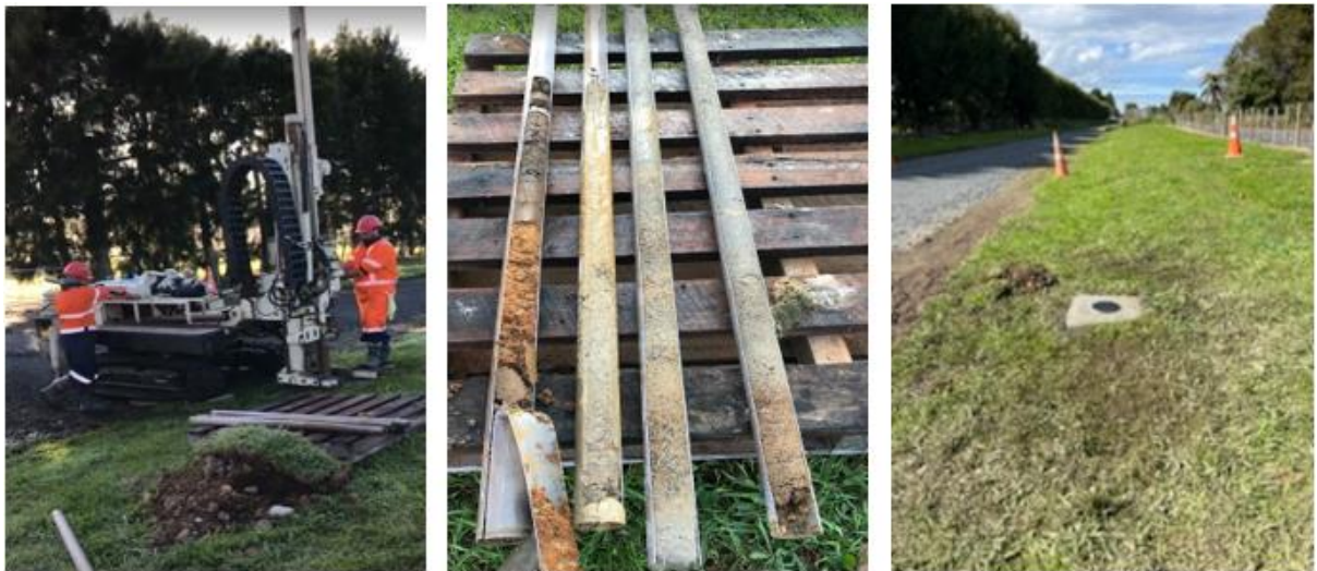
Matangi WWTP – Shallow piezometer monitoring bore installed via direct-push C.P.T rig.
